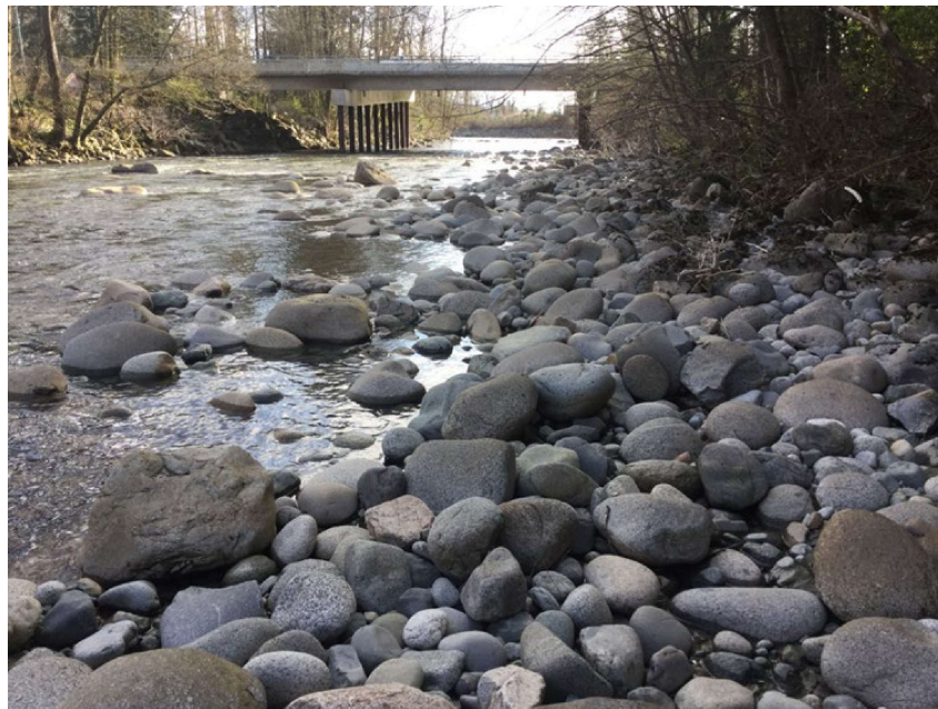
Figure 13. Looking downstream at SEY-DSSD06, April 3, 2020.
