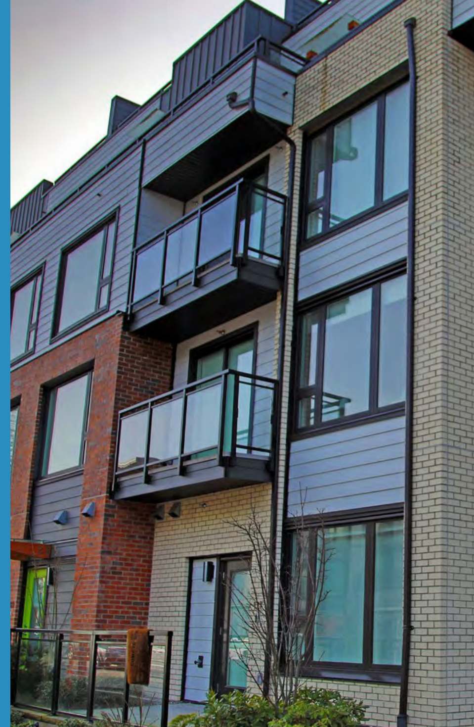
Roof runoff water is collected to support surface irrigation at The Trails Phase 1A development.
