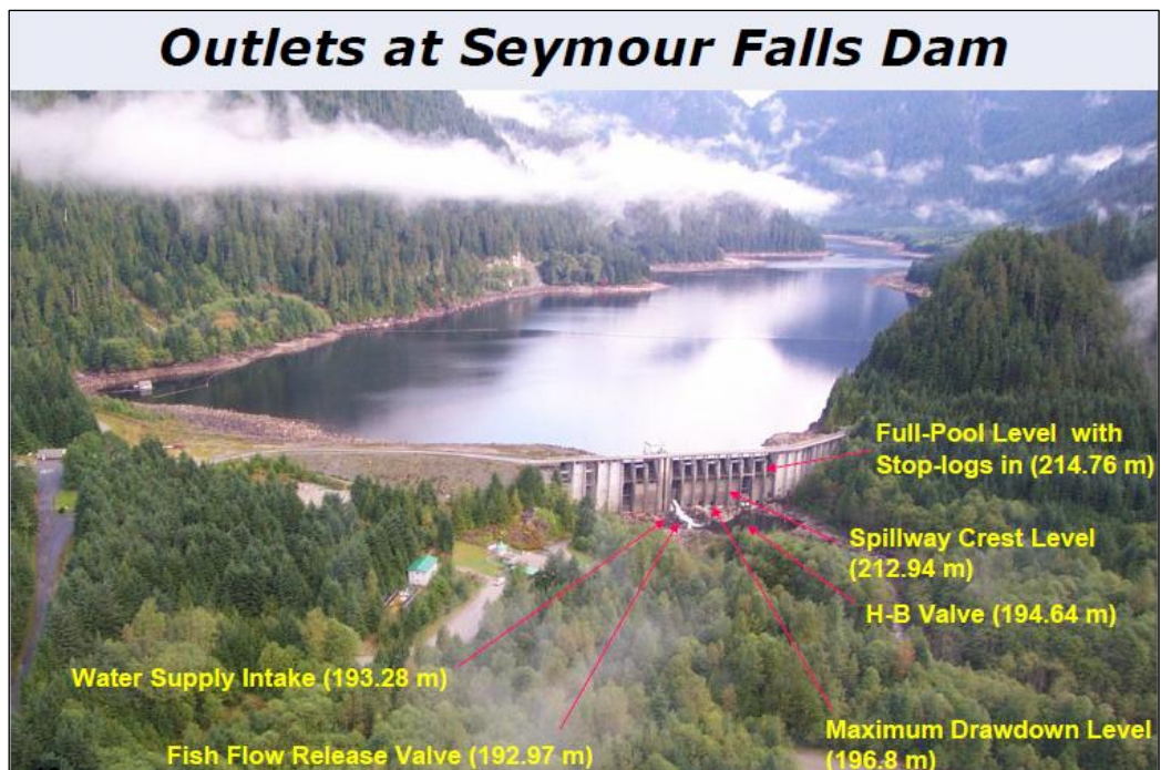
Figure 2-4 Outlets from Seymour Falls Dam
