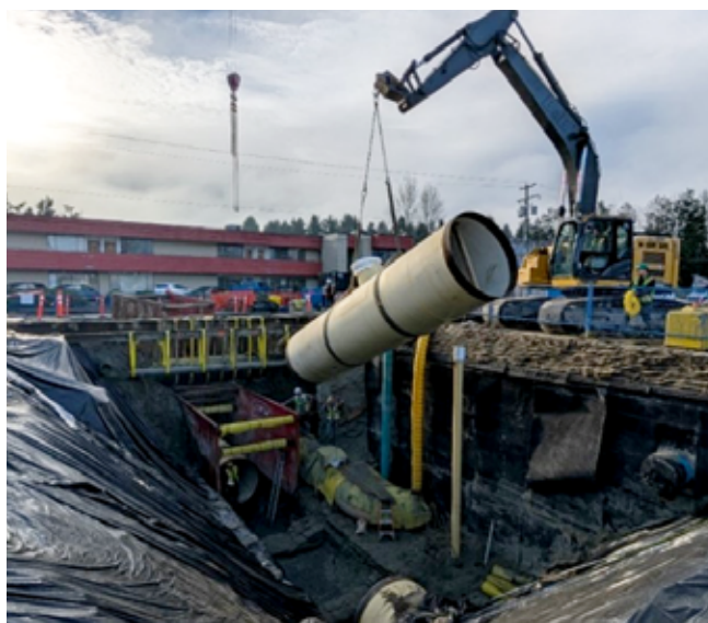
Figure 16: Kennedy Newton Water Main - Installation of 1.8m Diameter Water Main
