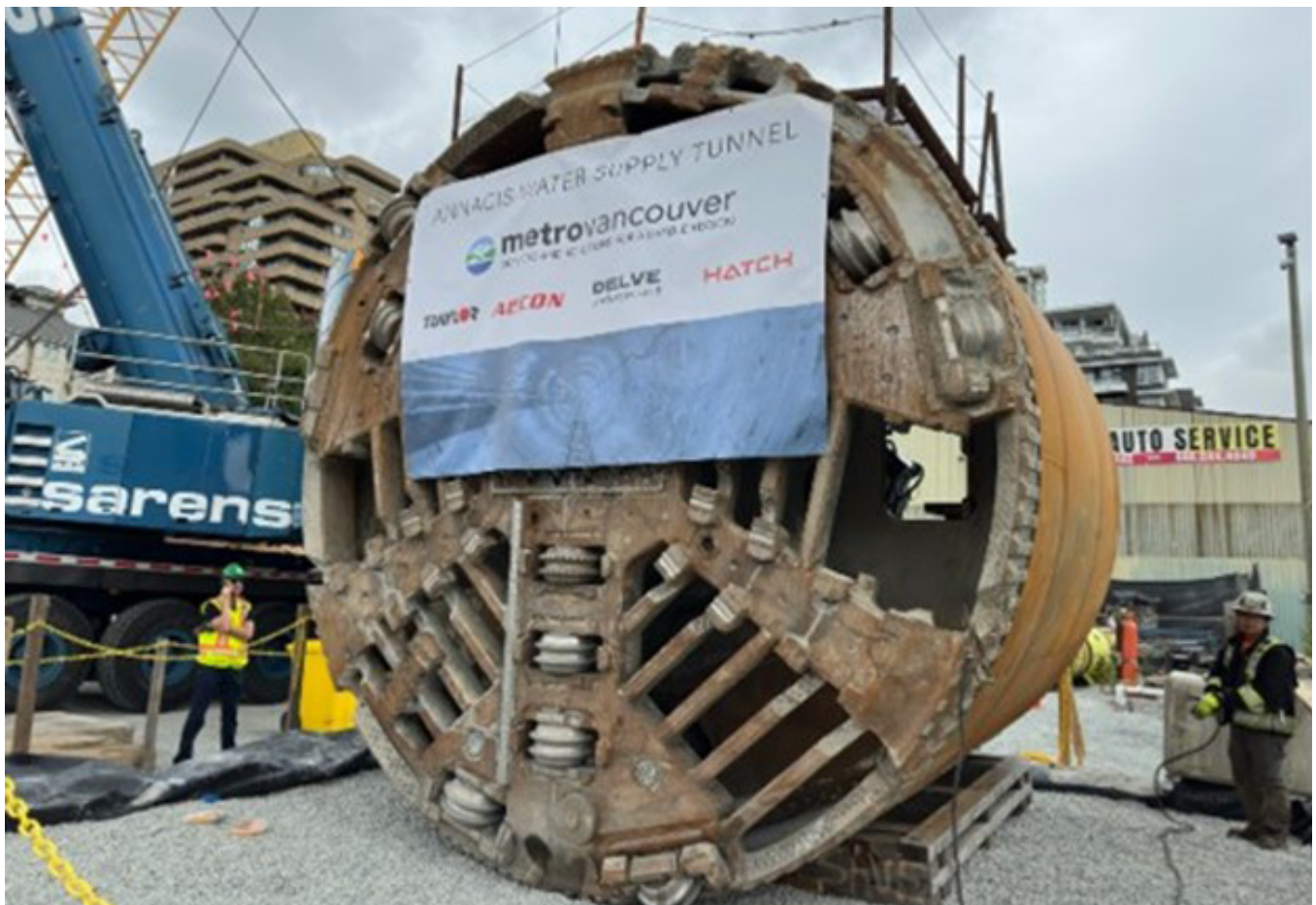
Figure 14: Annacis Water Supply Tunnel - Tunnel boring machine removal from north shaft
