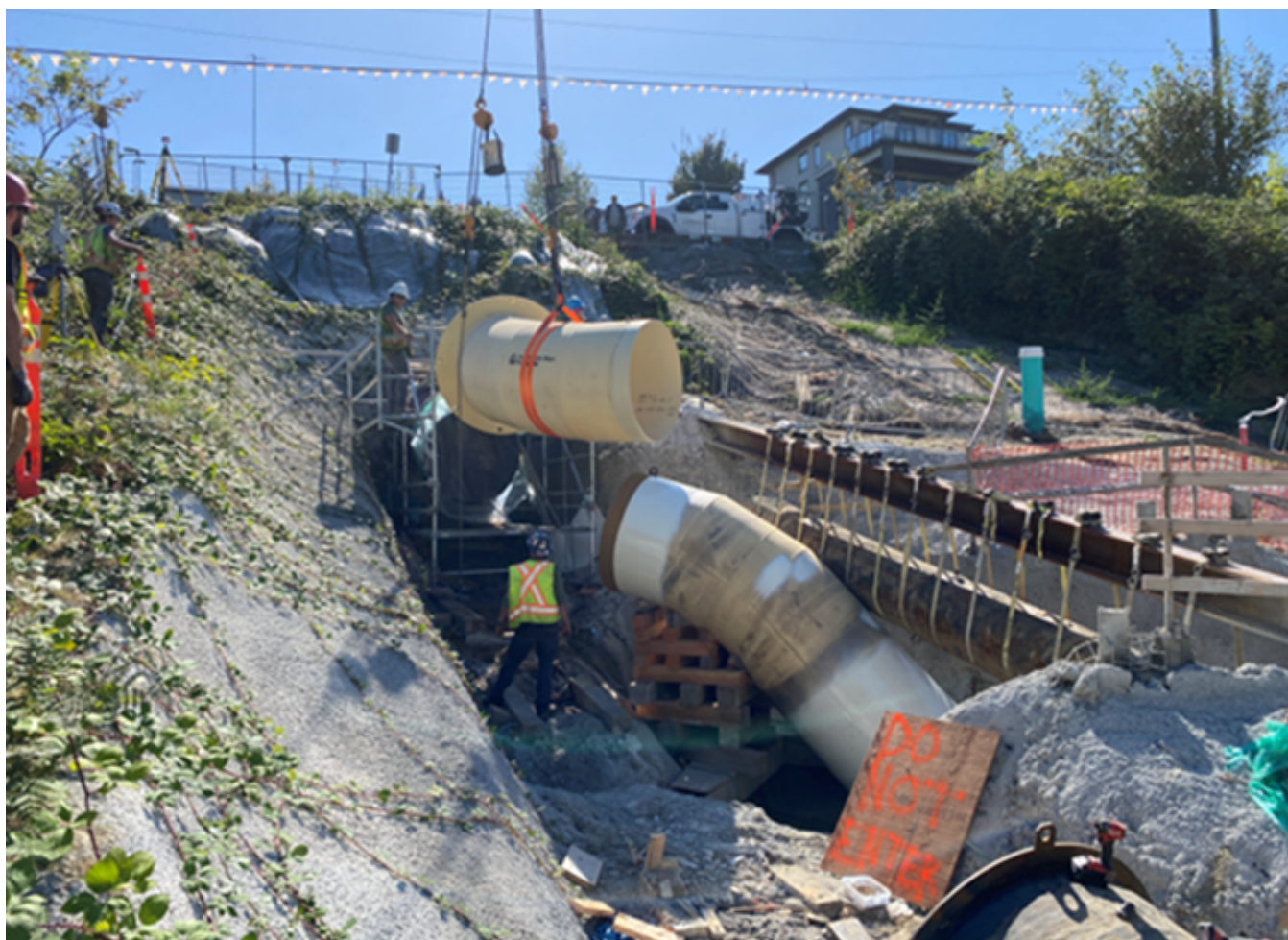
Figure 18: Second Narrows Water Supply Tunnel – Capilano Main No. 7 Tie-in
