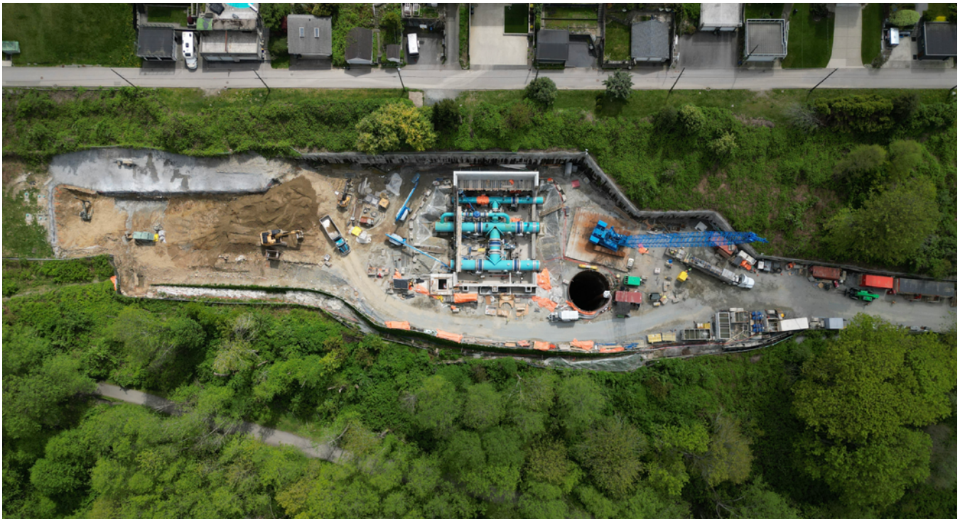
Figure 16: Second Narrows Water Supply Tunnel – valve chamber construction and south shaft
