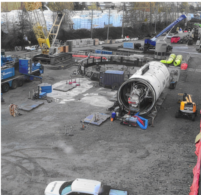
Figure 15: Annacis Water Supply Tunnel - Tunnel boring machine
