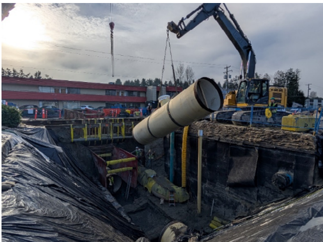
Figure 19: Kennedy Newton Water Main – Installation of 1.8m Diameter Water Main
