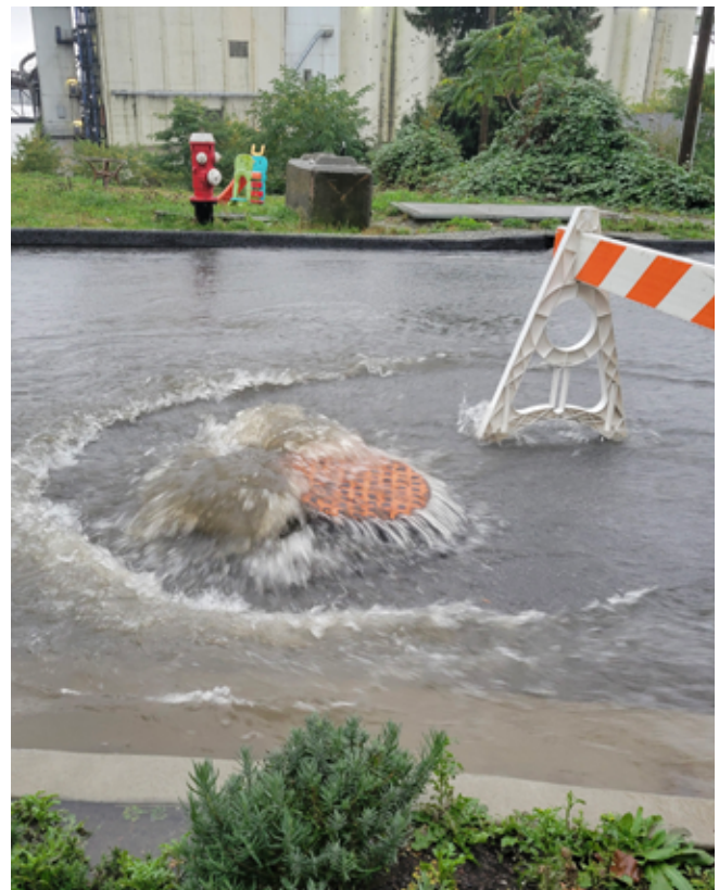
Storm sewer overflow
