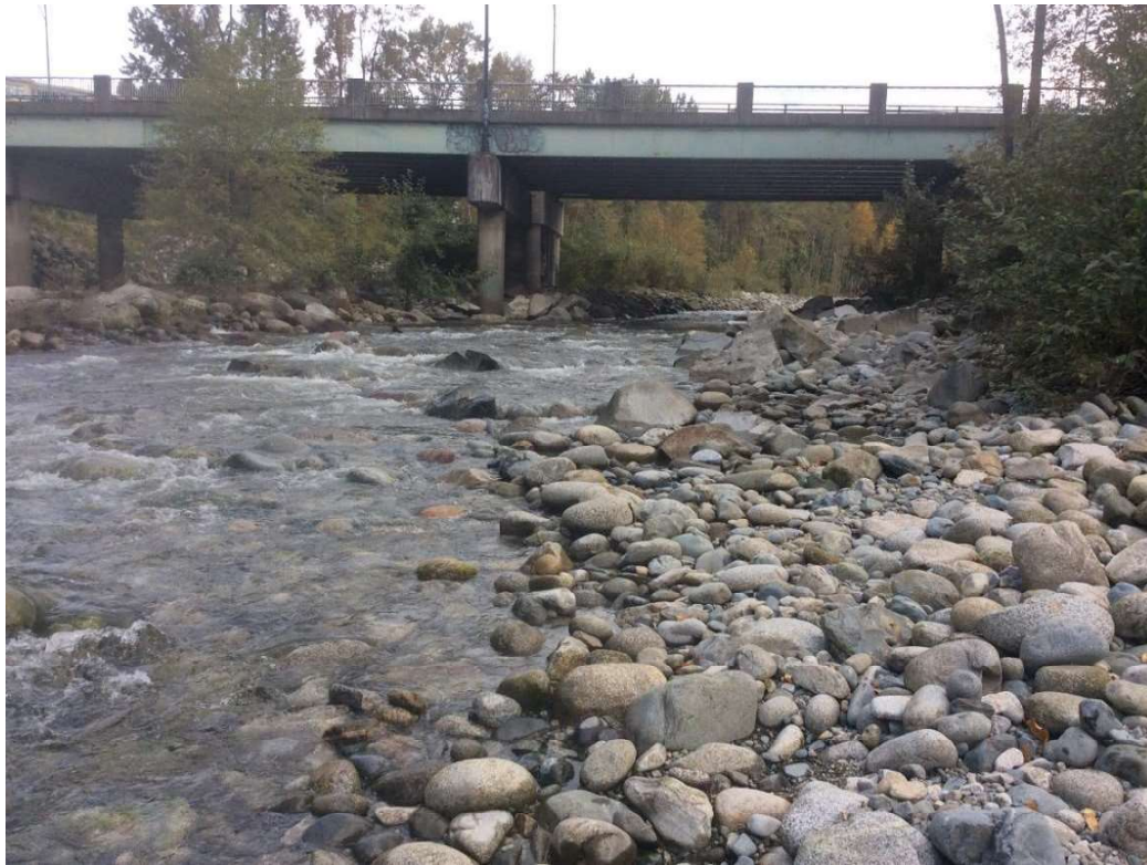
Figure 12. Looking upstream at CAP-DSSD07, October 1, 2019.
