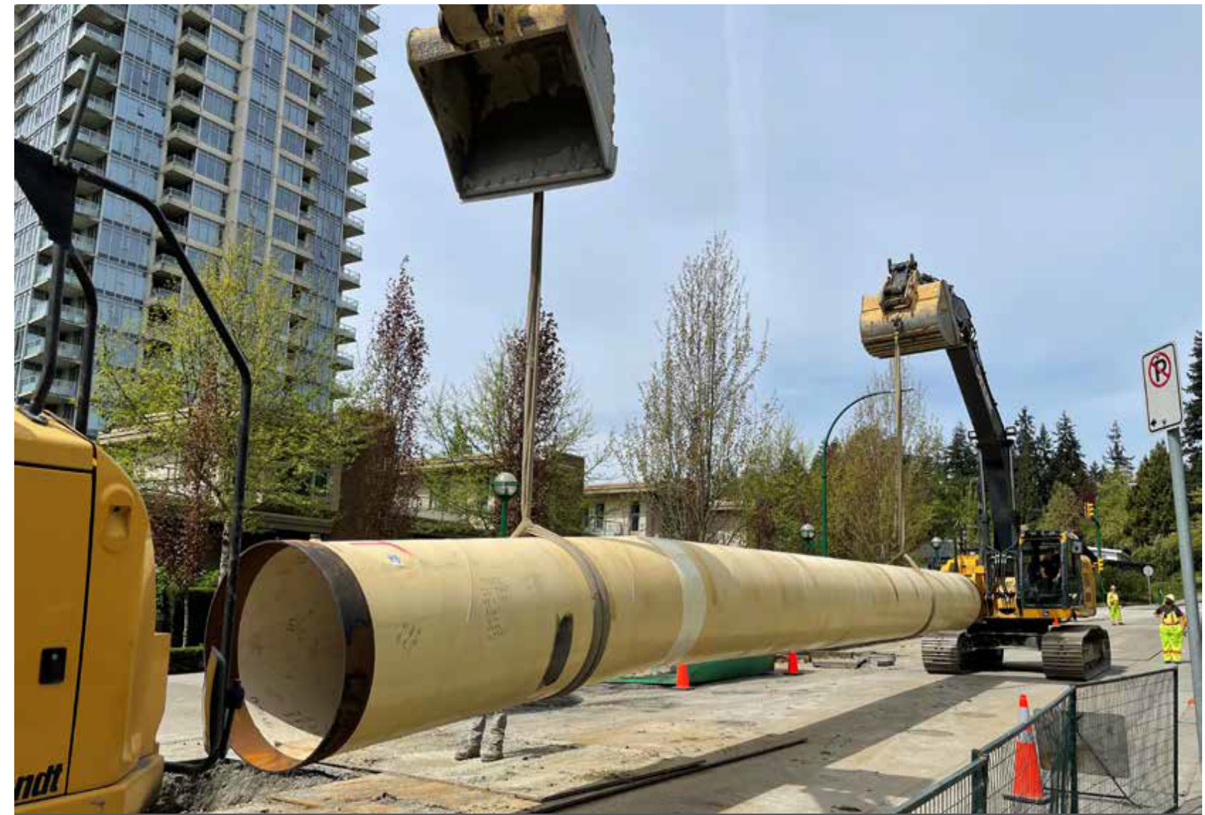
Using a crane to deliver the water main
