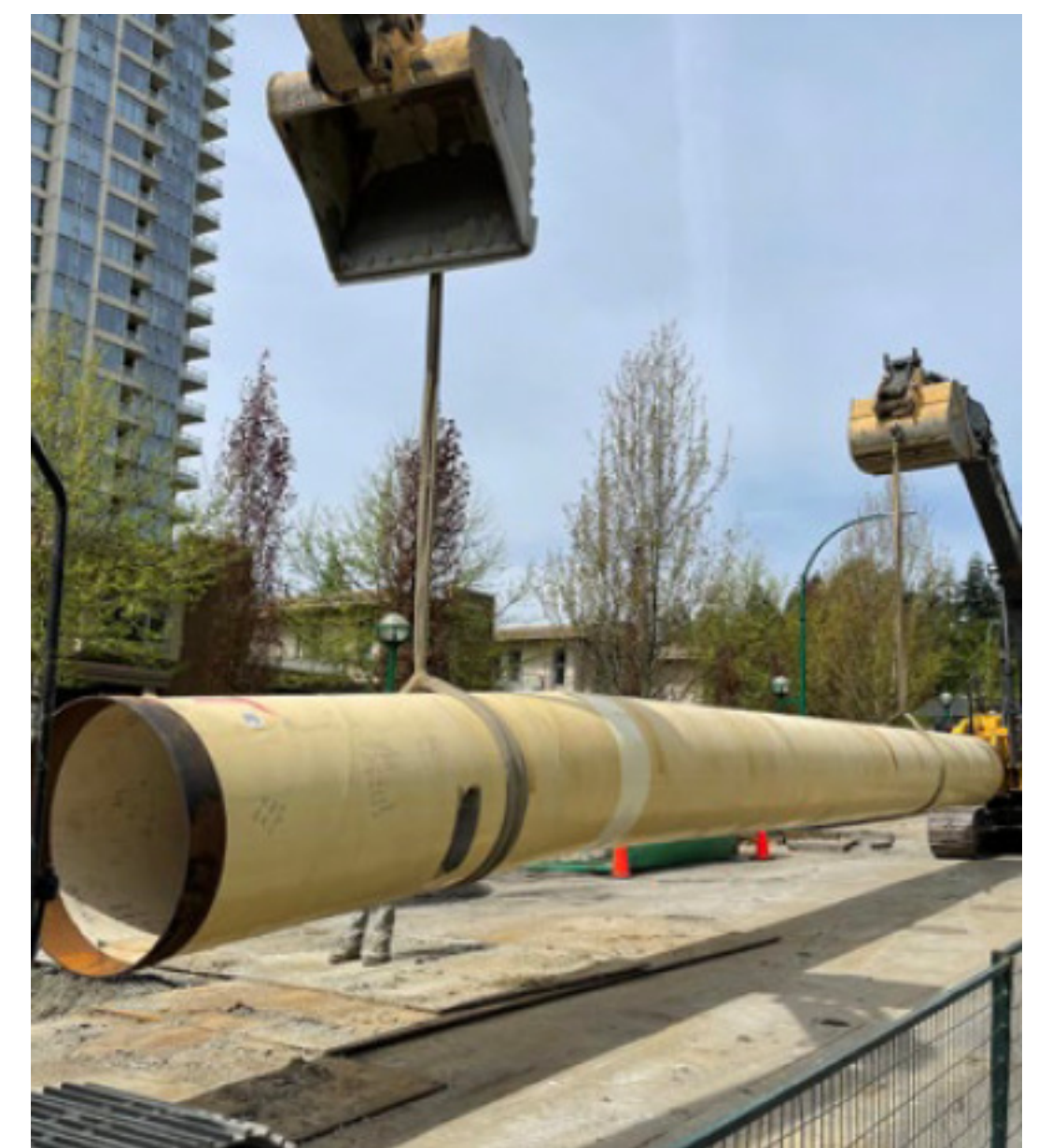
Construction of Central Park Water Main – Salisbury/18th Section
