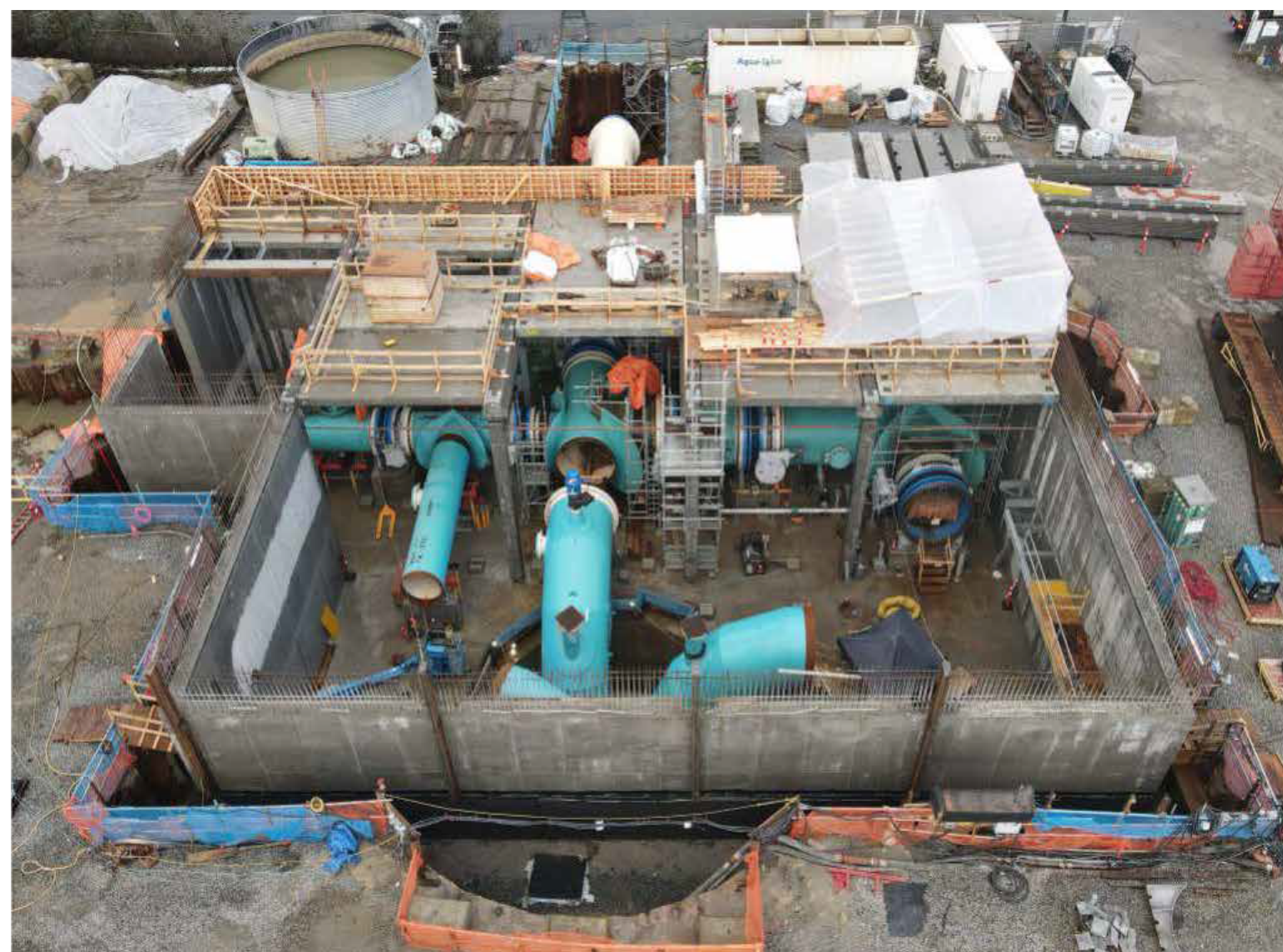
Constructing an underground valve chamber
