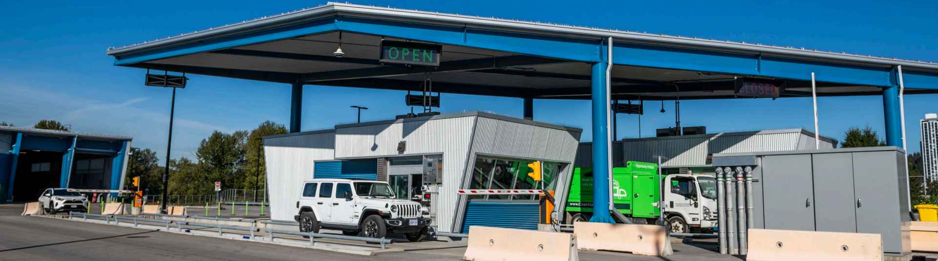
United Boulevard Recycling and Waste Centre Scale
