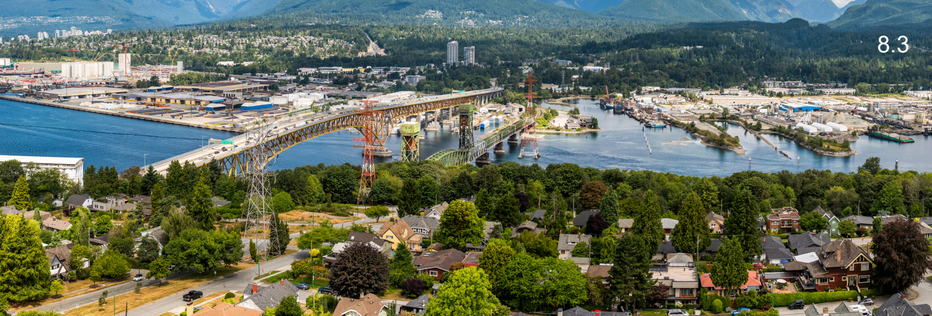
Overlooking Second Narrows Bridge
