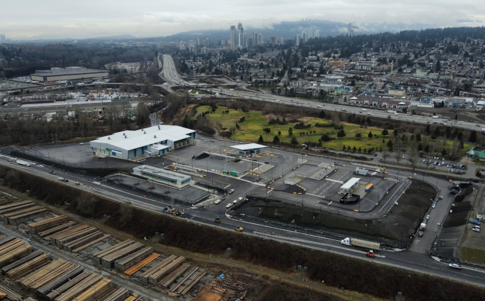
United Boulevard Recycling and Waste Centre 995 United Boulevard – Opened March 2022
