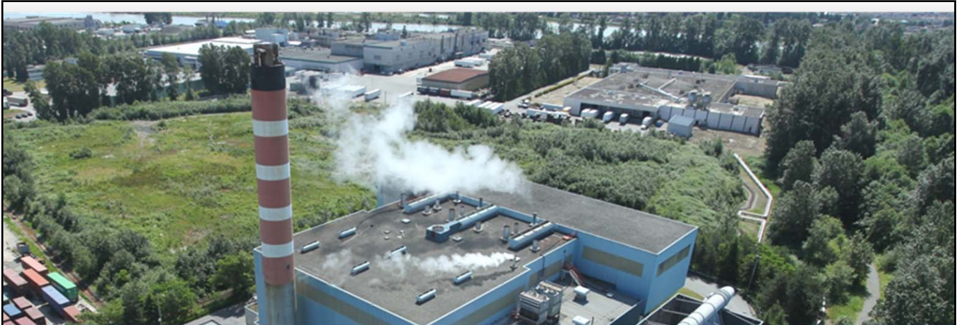
Photo: Waste-to-Energy Facility
