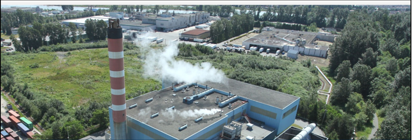
Photo: Waste-to-Energy Facility
