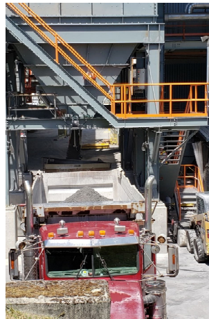
Loaded Fly Ash Trailers
