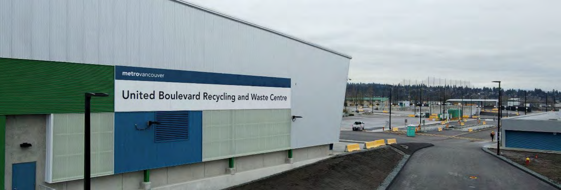
United Boulevard Recycling and Waste Centre
