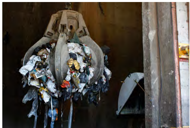
Garbage claw at the Waste-to-Energy Facility
