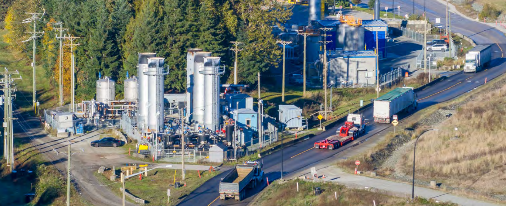
Vancouver Landfill flare station
