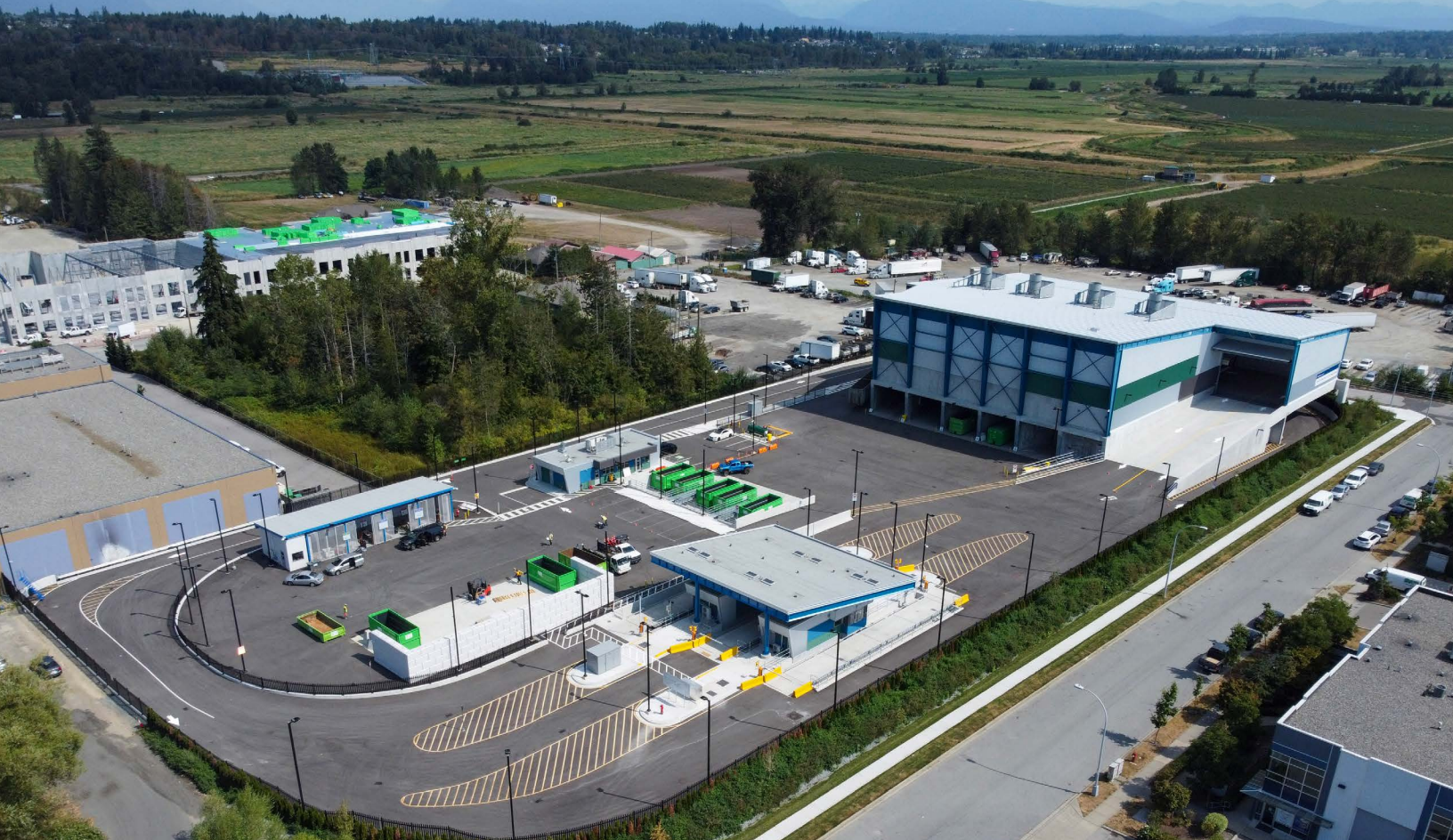
Central Surrey Recycling and Waste Centre
