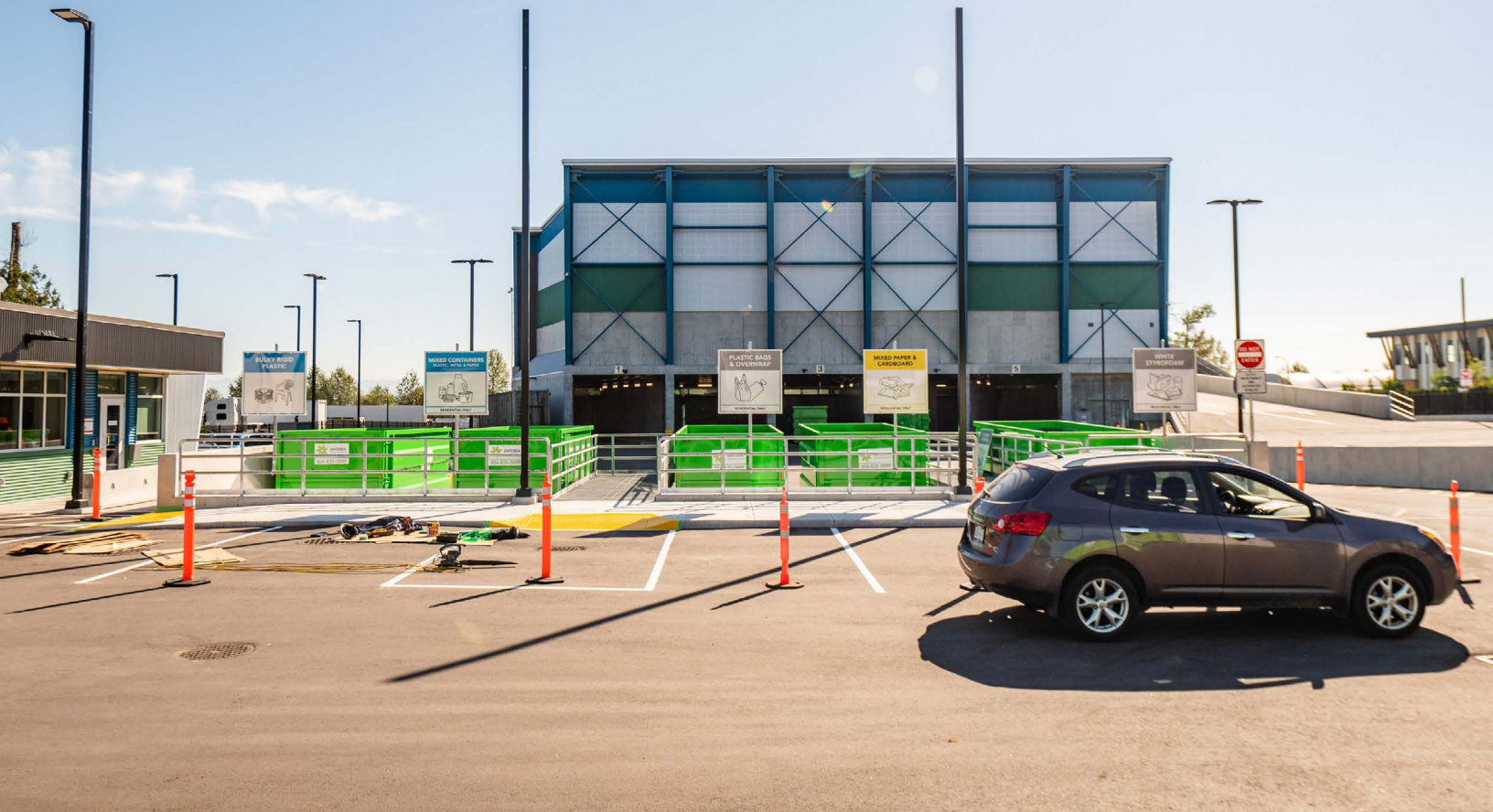
Central Surrey Recycling and Waste Center
