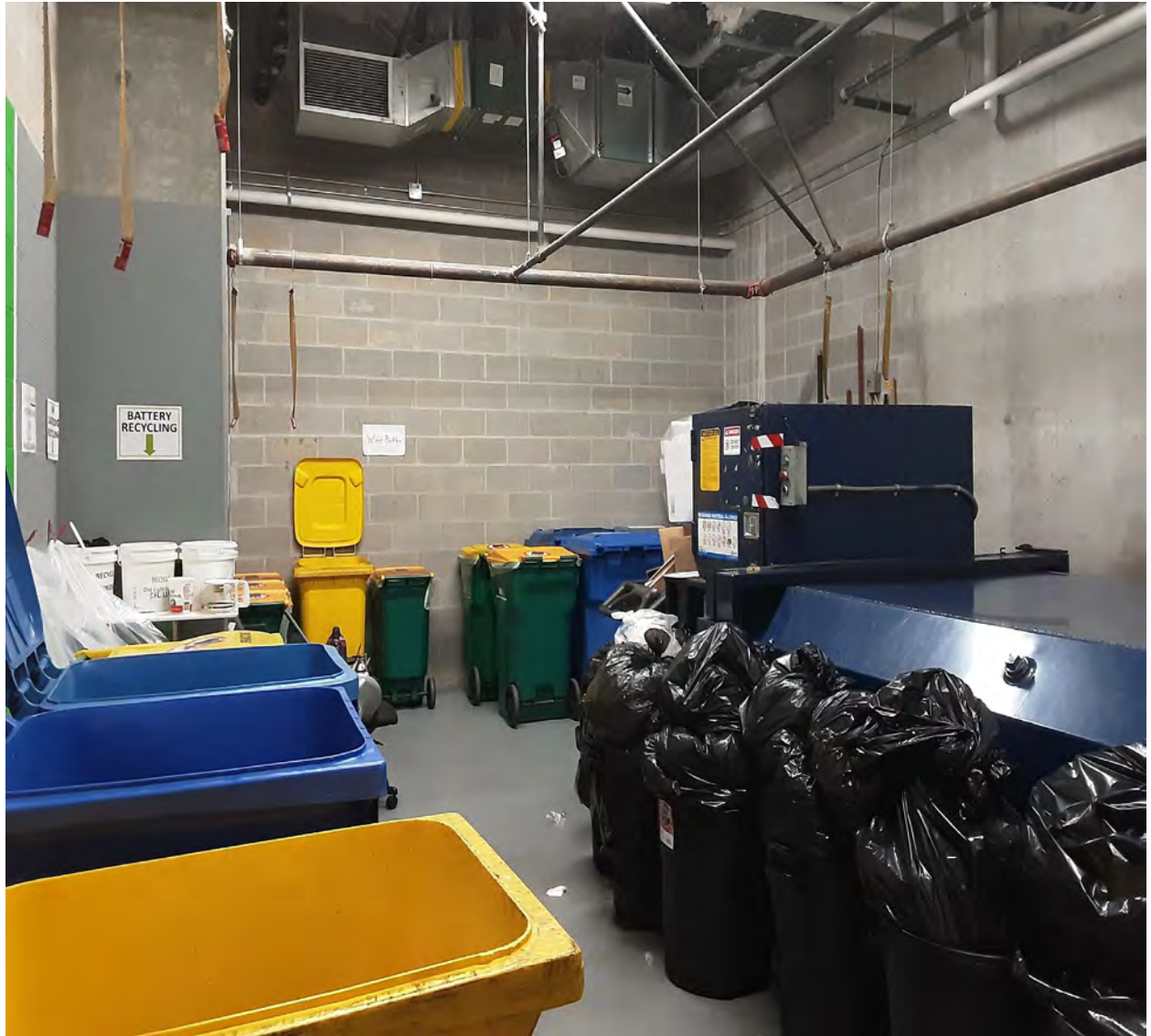
Photo 6-Garbage Room with Compactor at the site of Sample Number 37
