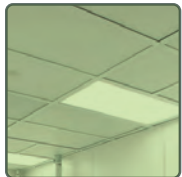
t-bar ceiling tiles drywall joints
