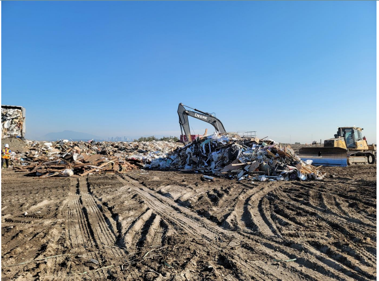
Photo 13: Excavator Spreading Sample Material
