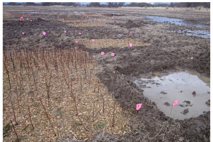
Live stakes installed through woodchip mulch covering at Bear Creek Park, Surrey.
