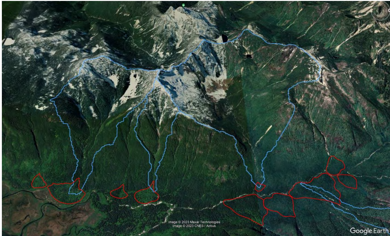
Figure B-3 Typical steep creek watersheds in Electoral Area A. Example above shows drainages in the Widgeon Valley. The approximate watershed boundaries are outlined in blue and fans are outlined in red. Google Earth May and July 2021 imagery.
