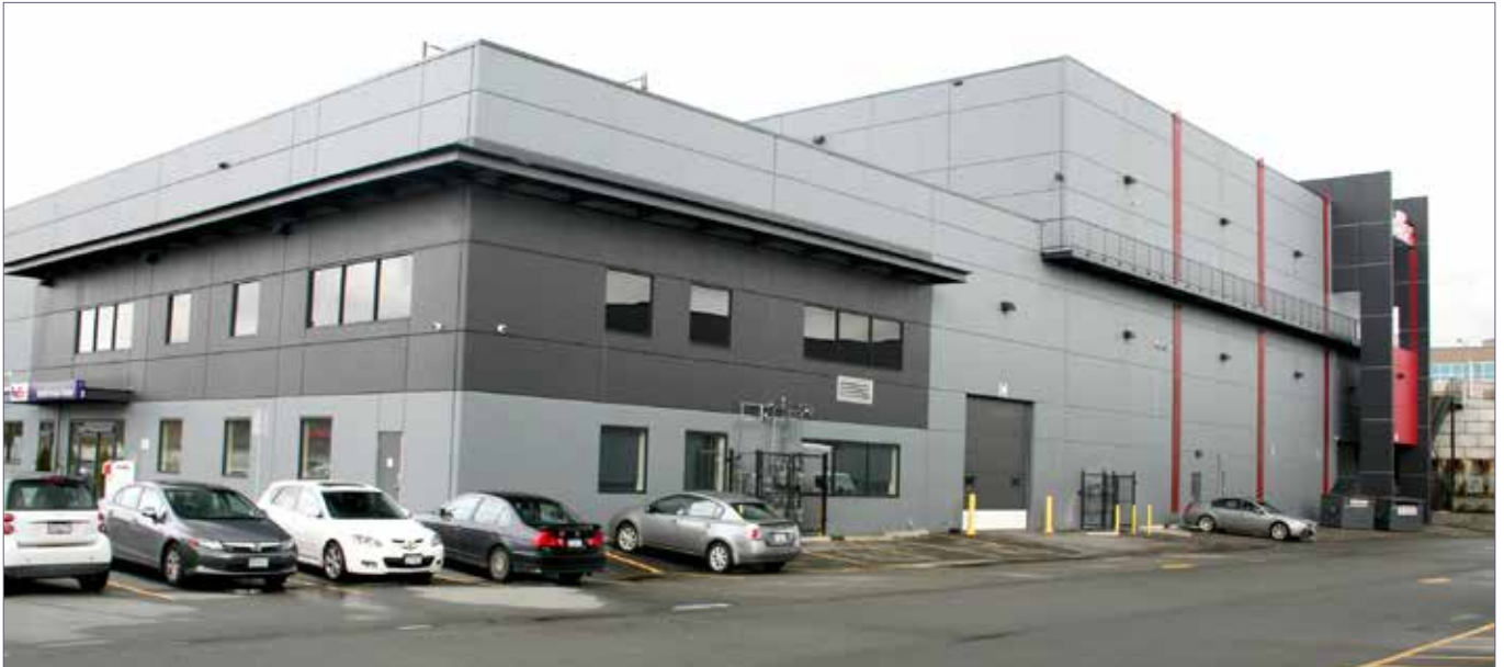
Multi-level industrial building in Surrey with light industrial use on ground floor and flex space and parking on upper floor. This is an example of a building with higher floor area ratio yet conventional site coverage.
