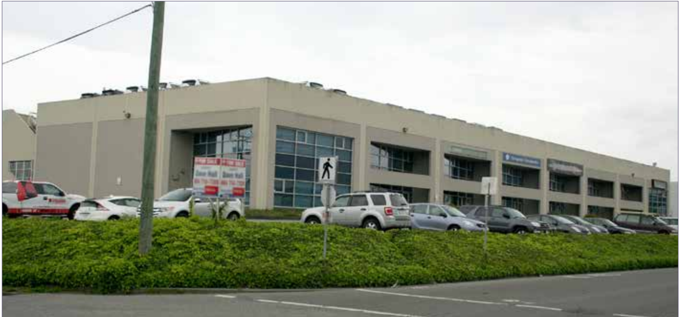
Photo of light industrial building with roof-top parking in South Vancouver with flex space for multiple tenants. Roof-top parking reduces the need for as much surface parking and can allow for greater building site coverage.
