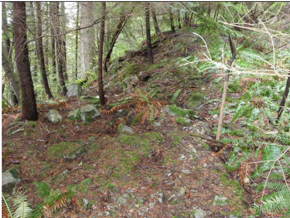
Photo 7. Unstable fillslope at WP194. View south. Note shovel stuffed into tension crack.
