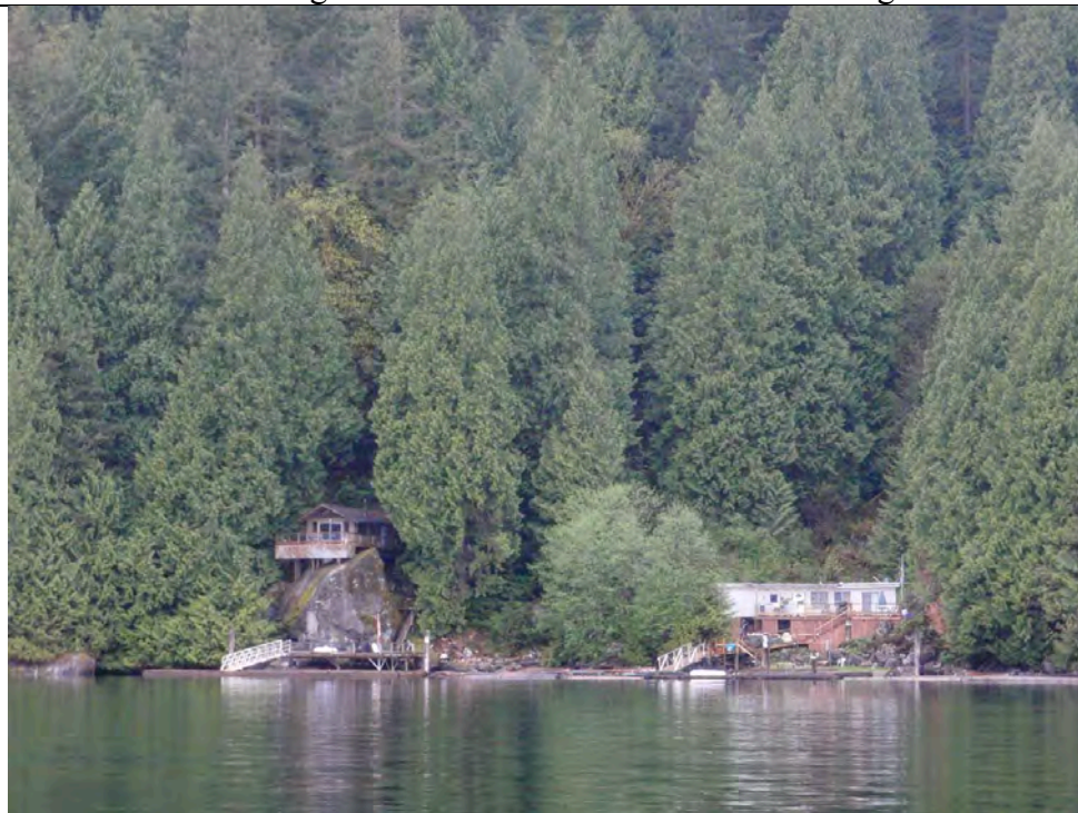
Photo 11. Lot 9 Cabin (left) built on large rockfall block below rockfall source area (Waypoints 205-206). Lot 8 cabin (right) was knocked off its foundation by 1990 debris slide. Lot 9 experienced a near miss, and was not affected because trees caused a jam and diverted the landslide toward Lot 8.
