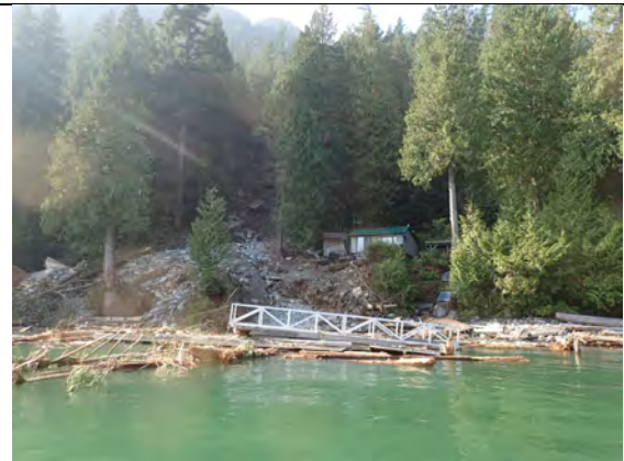
Photo 27. WP32. Lot 6. View west showing north (right) edge of debris flow track which tore porch off cabin. Cabin otherwise intact.
