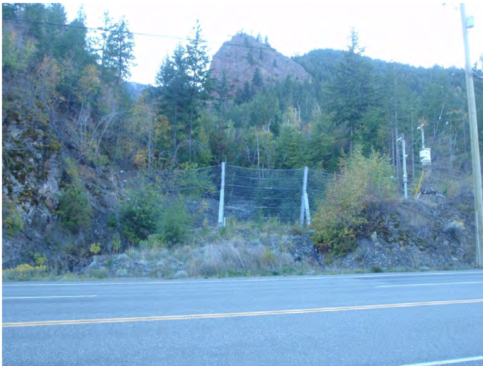
Figure 4. Debris fencing installed to protect Highway 1 just east of Lytton.
