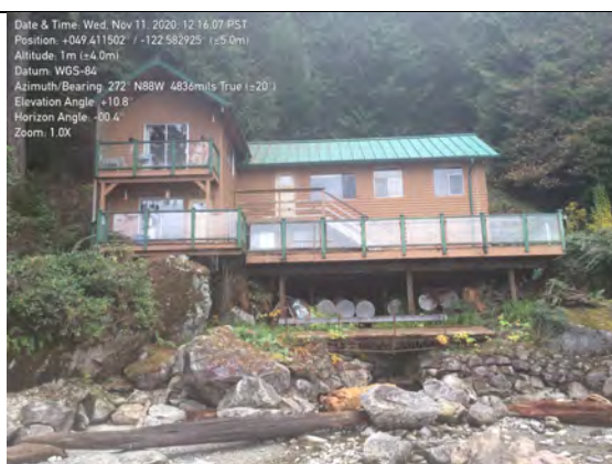
Photo 32. Cabin on Lot 10. The 1990 debris flow just missed (<10 m) the north (right) side of this building. Note the box culvert & creek beneath the cabin.
