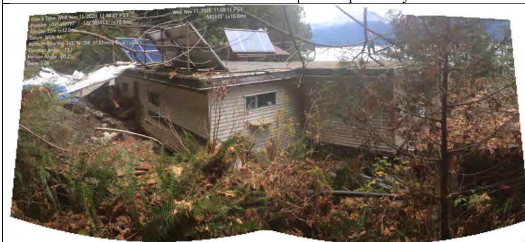
Photo 30. WP97. Lot 8. Back of cabin affected by 2020 afterflow slurry, accumulated to 1 m depth. In 1990, this cabin was knocked off its foundation and then reset in its present position (see Appendix 2)
