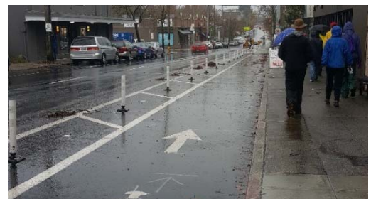
Figure 14: Phasing in a separated cycle track is one TDM strategy Seattle DOT and King County Metro are using to support the implementation of a new BRT-light service along the Roosevelt Corridor. The cycle track replaced one parking lane, rebalancing the road way to be more multi-modal and to improve non-motorized access to transit.
