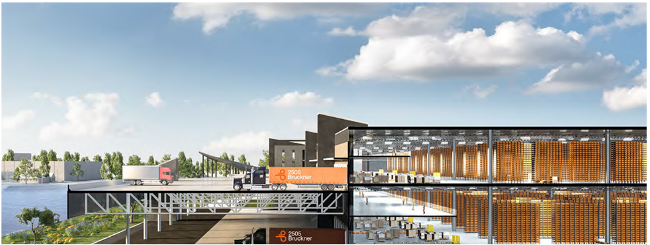
Truck loading on the second floor ensures the efficiencies associated with ground level access.
