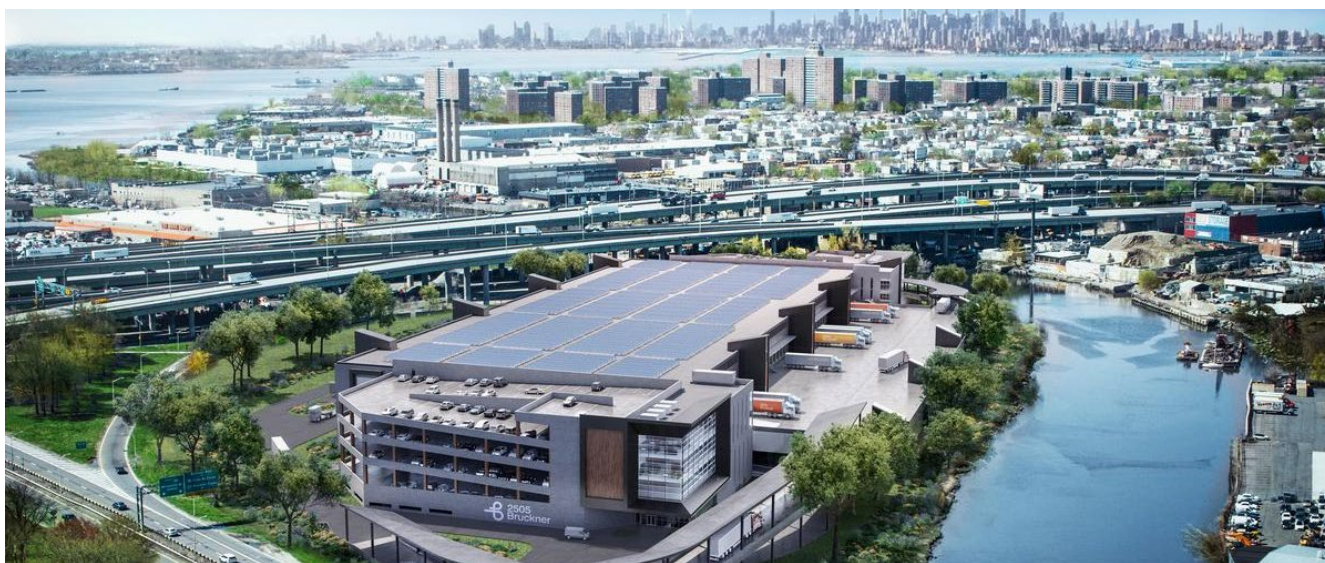
2505 Bruckner Boulevard will feature 2 levels of large-format industrial space with direct 2 nd floor truck access through a ramp.
