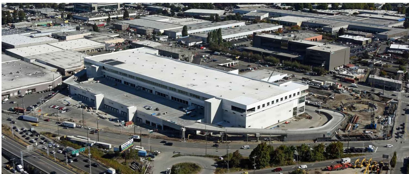
Prologis' Georgetown development in the City of Seattle was North America's first modern multi-storey industrial development.
