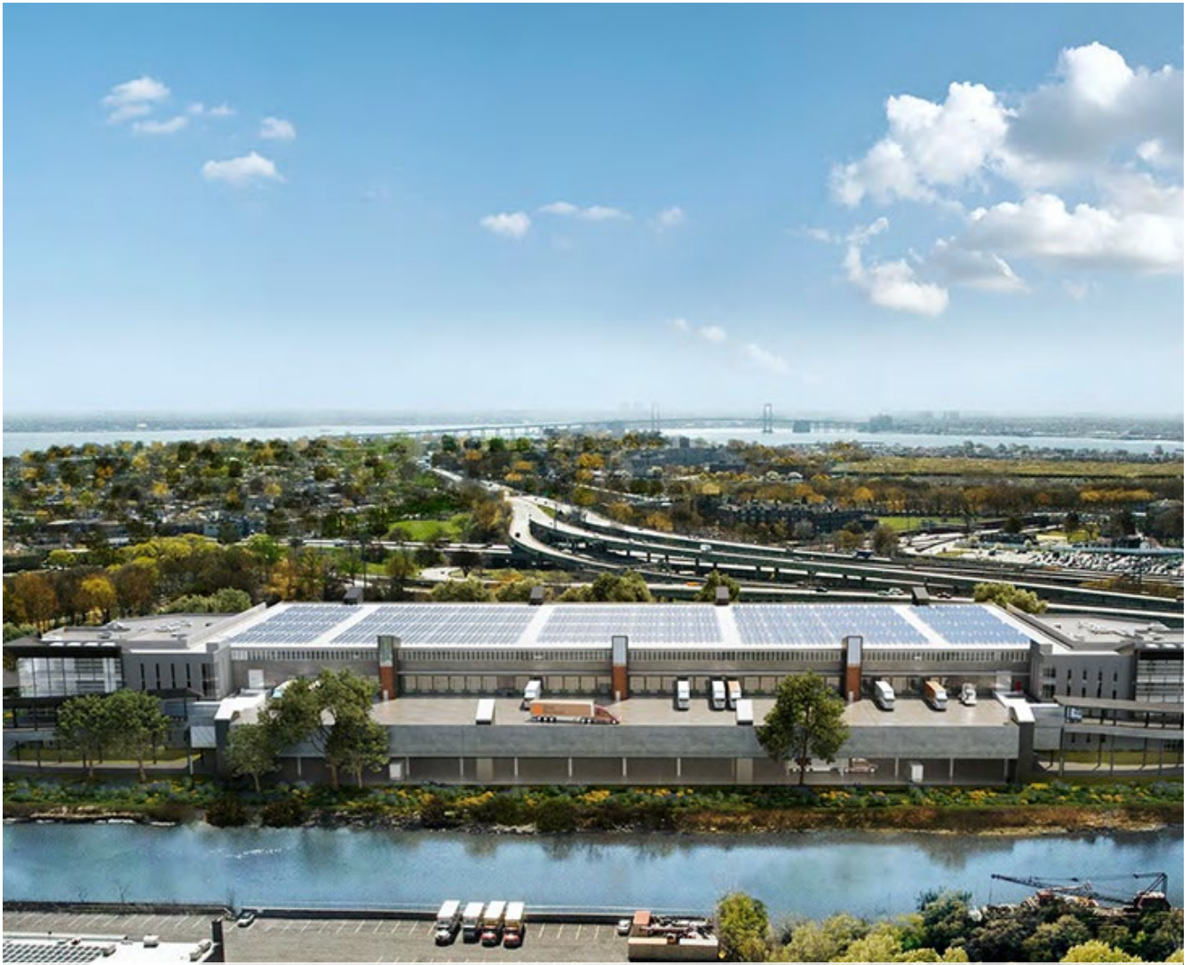
The site is strategically located within an extremely dense trade area providing a population of 9.4 million within 15 miles.
