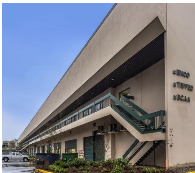
3030 Beta Avenue in Burnaby benefited from a sloped site to provide two levels of truck access without building a ramp.
