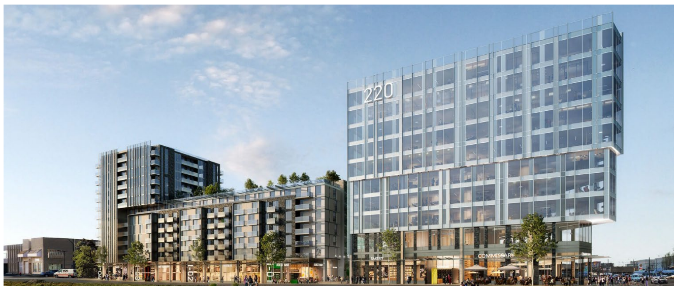
Archetype is the first mixed-use project in Vancouver to include strata commercial/industrial space with rental residential.
