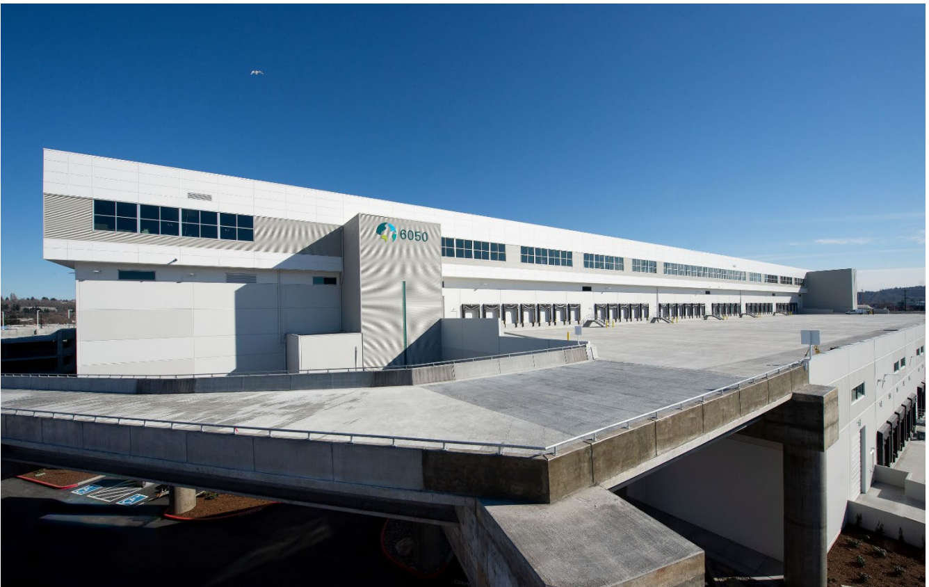
The construction of a ramp suited to accommodate large North American sized trucks added significant costs to the development.
