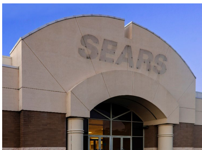
Vacant anchor tenants are beginning to be repurposed by companies such as Amazon for fulfillment centres.
