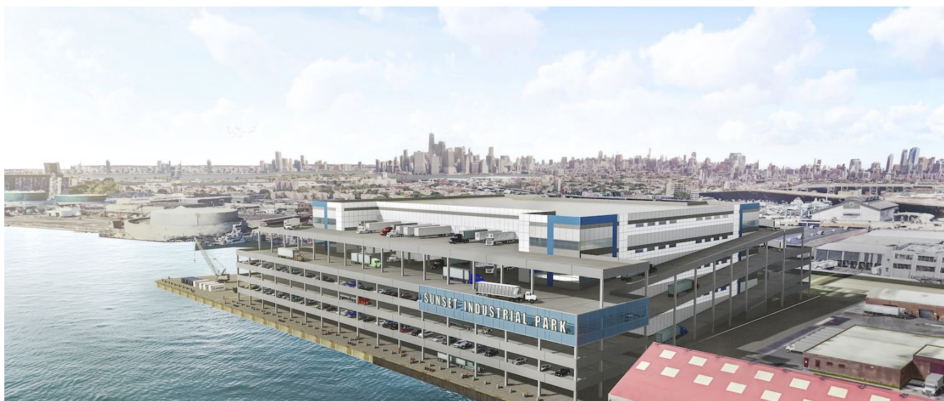
The four-floor Sunset Industrial Park will be the largest multi-storey, large-format industrial development in North America.
