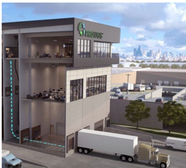
Above ground loading via freight elevators is often perceived as undesirable even though it can be quite efficient.
