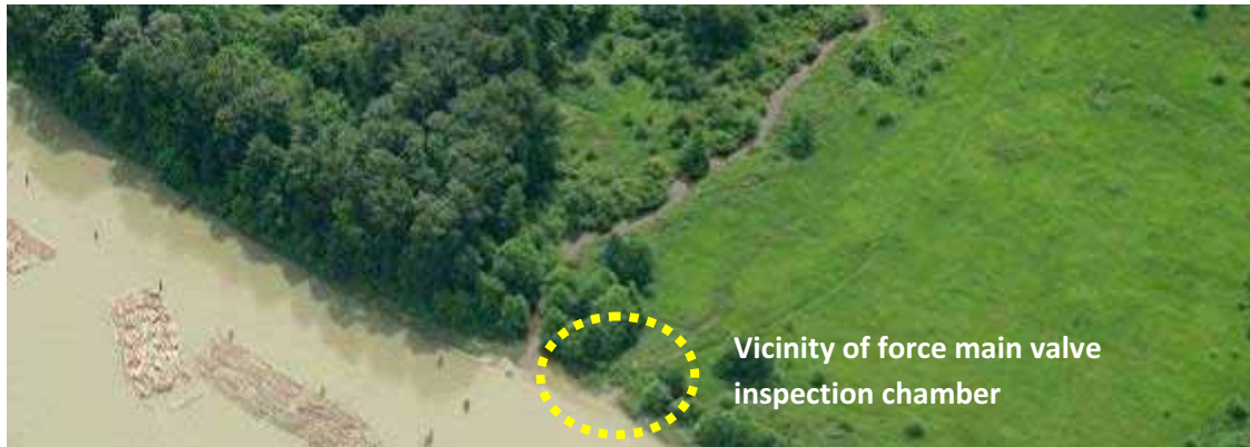
Figure 6: Force Main Valve Inspection Chamber
