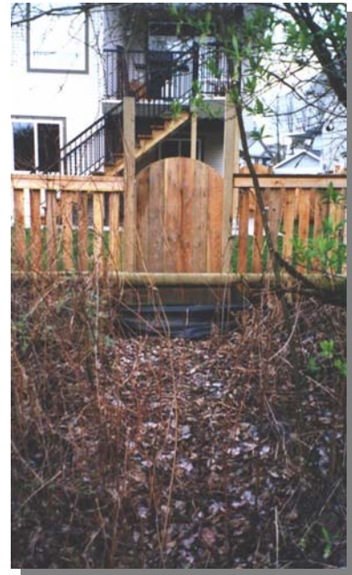
Encroachment on park boundary
