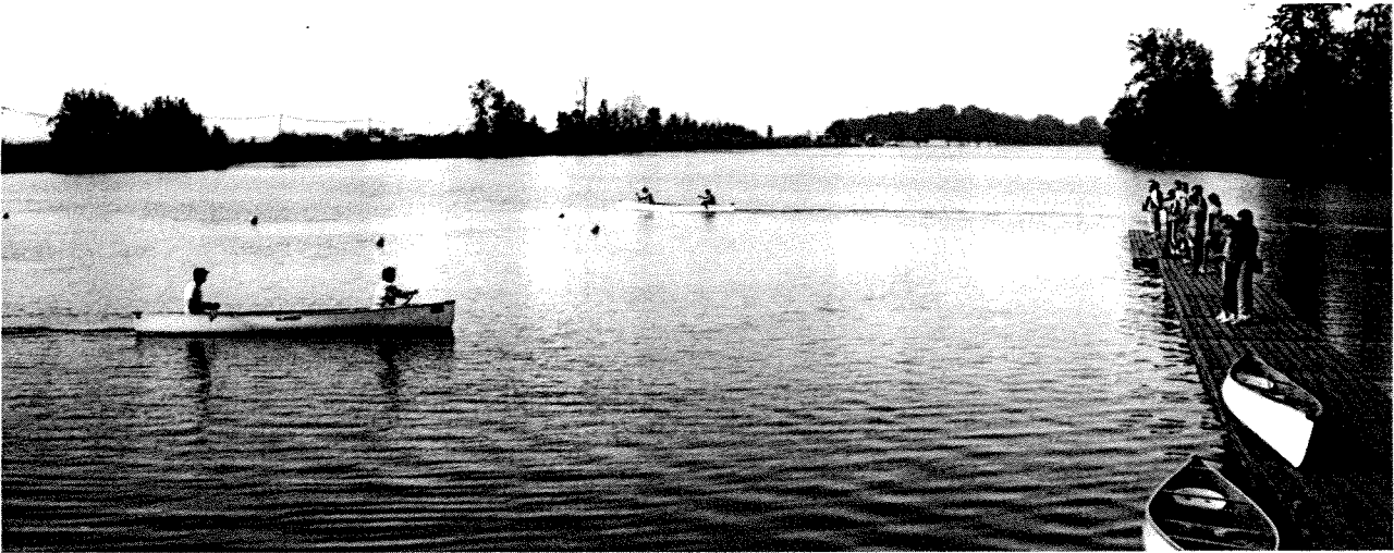
CANOEING IN DEAS SLOUGH AND THE RECENTLY INSTALLED FLOAT
