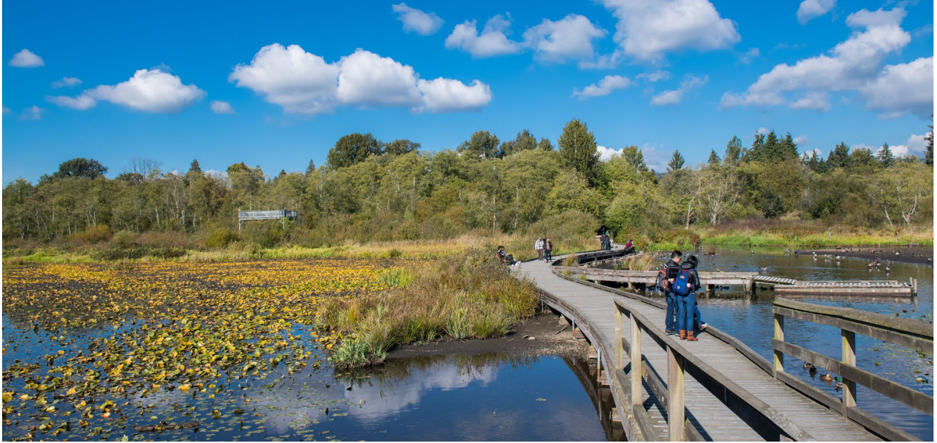
PIPER SPIT BOARDWALK AND VIEWING TOWER, BURNABY LAKE REGIONAL PARK
