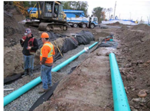
Infiltration trench being installed at Mountain Equipment Co-Op in North Vancouver, BC. (Photo Credit: Kerr Wood Leidal Associates Ltd.)
