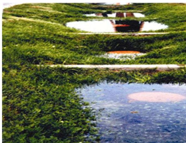
Swale with check dams in operation.
