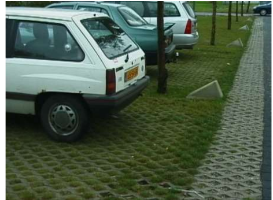
Concrete grid paving parking lot, Netherlands (Photo Credit: Lanarc Consultants Ltd.)
