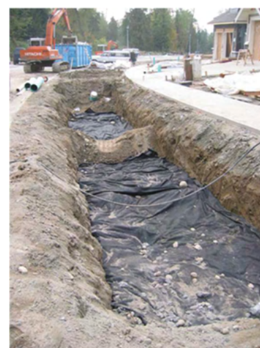
Trench installation, showing filter cloth wrap, and showing trench dam of native material between infiltration trench 'cells'.
