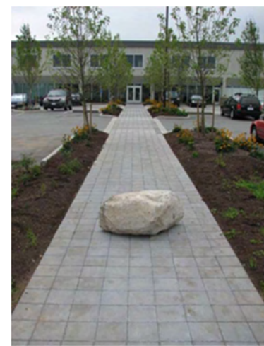
Permeable paver walkway, Mountain Equipment Co-op, Surrey, BC.
