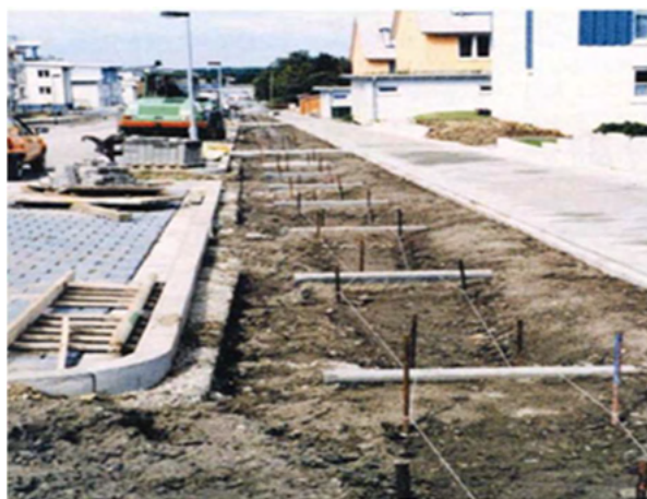
Swale with check dams under construction.
