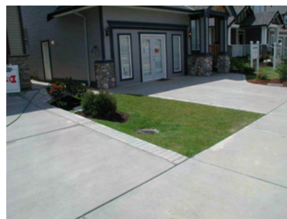
Completed single family lot infiltration trench completed; lawn basin is the only visible indication that it is there.
