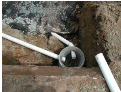
Single family lot infiltration trench being installed in East Clayton development, Surrey, BC.
