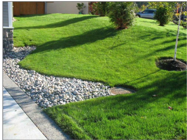
Disconnected roof leader and absorbent landscape in Maple Ridge.
