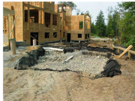
Infiltration trench can be in any plan shape – the photo shows a rectangular infiltration trench under construction at a single-family subdivision in BC.
