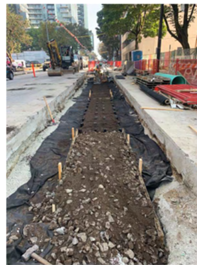
Silva Cell (proprietary) and structural soil installed adjacent to one another, Vancouver.
