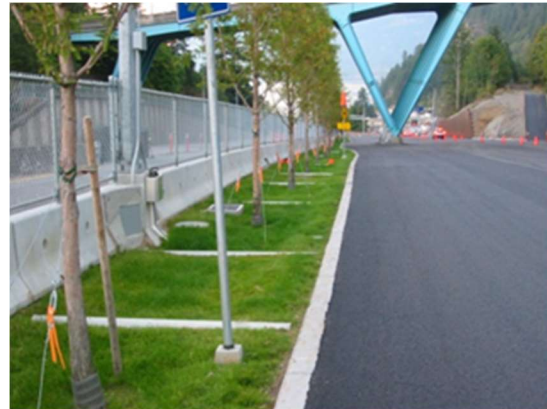
Flush curb draining to terraced grassed swale at Horseshoe Bay Ferry Terminal, West Vancouver, BC
