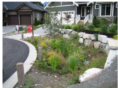
Roadside rain garden with flat panel curb and shrub and herbaceous plantings in Thunderbird subdivision, Squamish, BC. (Photo Credit: Kerr Wood Leidal Associates)
