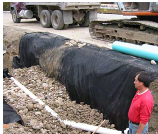
Perforated pipe over drain rock reservoir at infiltration trench under construction in Maple Ridge.
