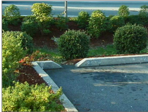
Drainage from parking area to landscape. (Photo credit: Lanarc Consultants Ltd.)
