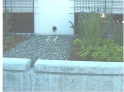
Flow-thru planter – a formal-shaped rain garden that provides water quality treatment and limited flow attenuation – adapted to a near-building location at Buckman Terrace in Portland, Oregon. (Photo Credit: Lanarc Consultants Ltd.)
