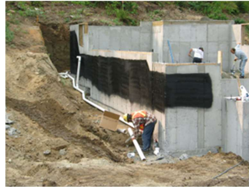
Infiltration facilities near urban structures should only be installed in neighbourhoods that have footing drains or other methods to protect basements from flooding.
