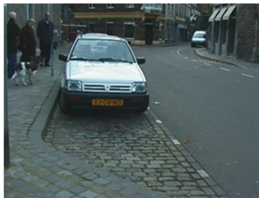
Permeable unit paving streetside parking in the Netherlands.
