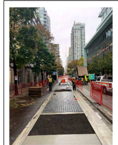
Tree pit and pavers over soil cells. (Photo Credit: City of Vancouver.)
