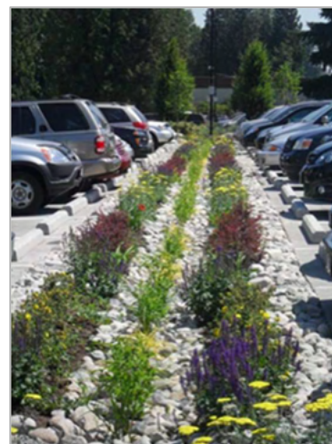
Planted and rock-lined Infiltration Swale, Rocky Point parking lot, Port Moody, BC.
