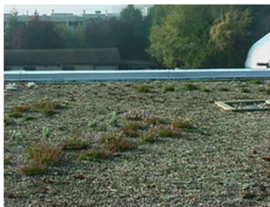
Newly planted extensive green roof showing plant-free zones at drain and edges – White Rock Operations Building.
