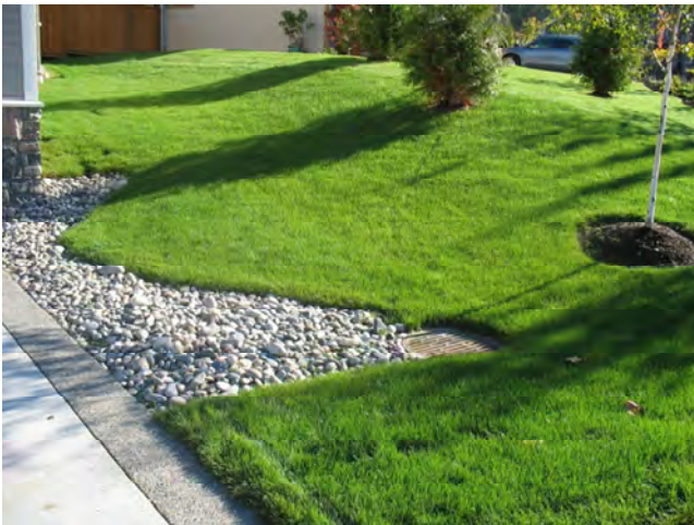
Disconnected roof leader and absorbent landscape in Maple Ridge, BC.
