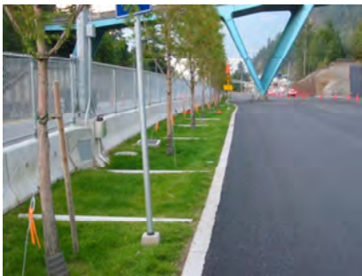
Flush curb draining to terraced grassed swale at Horseshoe Bay Ferry Terminal, West Vancouver, BC.
