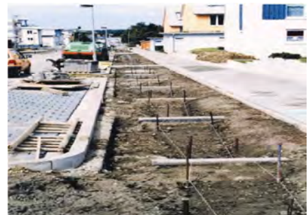
Swale with check dams under construction.
