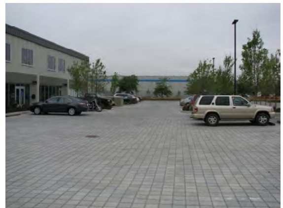
Permeable unit paver parking lot at Mountain Equipment Co-Op, Surrey, BC.
