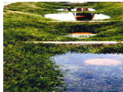
Swale with check dams in operation.
