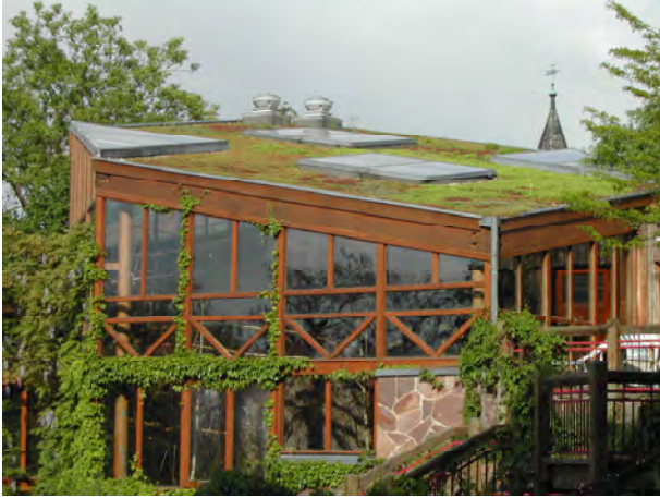
Extensive green roof – Halle Zoo, Germany
