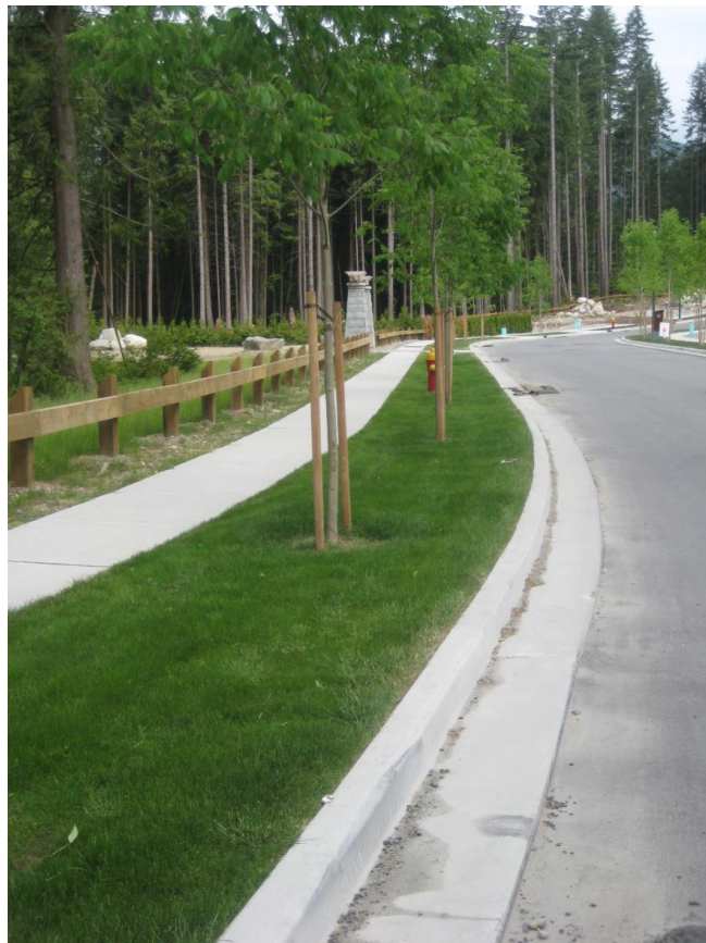
Photo 7: A Roadside Infiltration Trench
