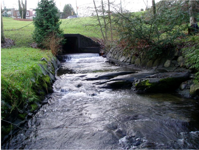
Photo A3 - A higher gradient stream in an urban area (Still Creek, Vancouver, BC). The creek flows out of a large culvert. Stream banks are armoured and bed morphology has been altered by limited sediment supply.
