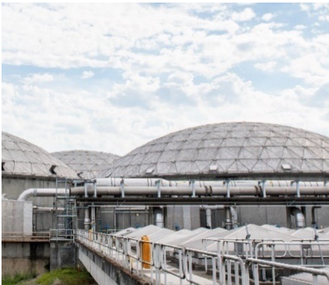
Annacis Island Wastewater Treatment Plant trickling filters
