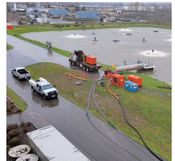
Northwest Langley Wastewater Treatment Plant equalization pond with temporary pumping to emergency storage – November 2021 atmospheric river
