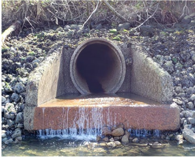
Willingdon #1 combined sewer overflow outfall – Burnaby
