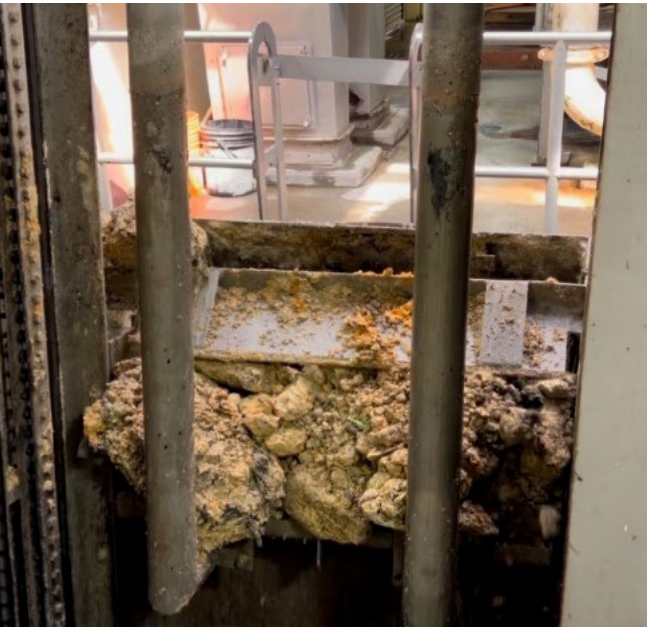
Influent bar screen clogged with “fatbergs” at Lulu Island Wastewater Treatment Plant
