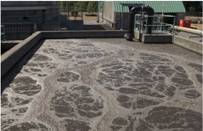
Northwest Langley Wastewater Treatment Plant – aeration tank
