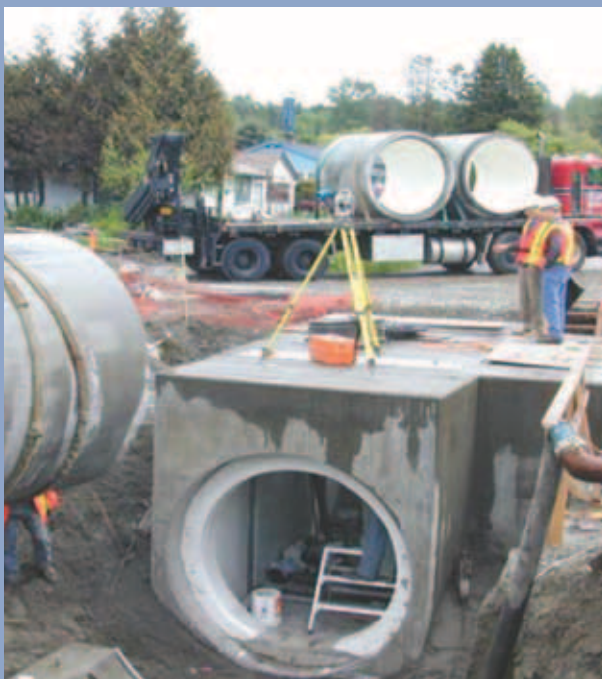
Installing Metro Vancouver trunk sewers, South Surrey.
