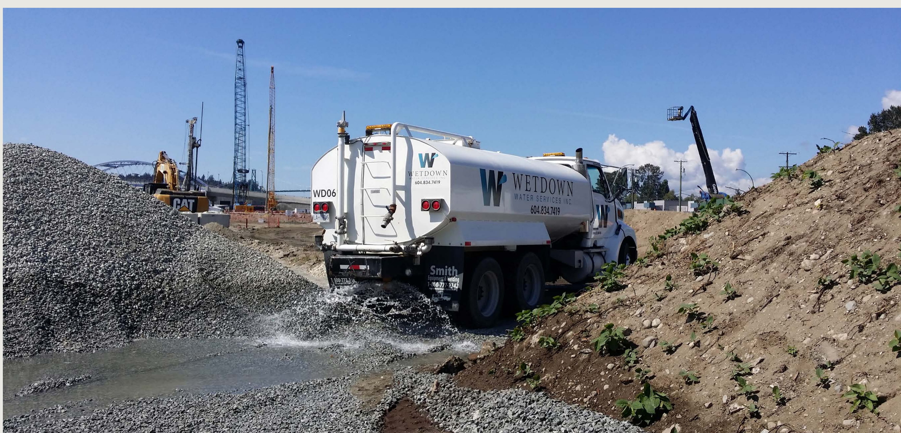
Metro Vancouver implementing dust control measures
