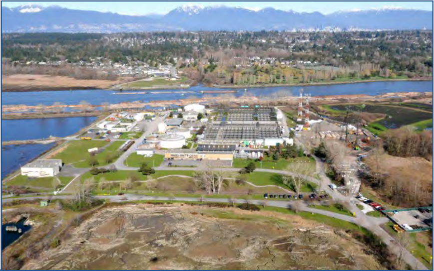
Iona Island Wastewater Treatment Plant
