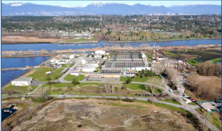
Iona Island Wastewater Treatment Plant
