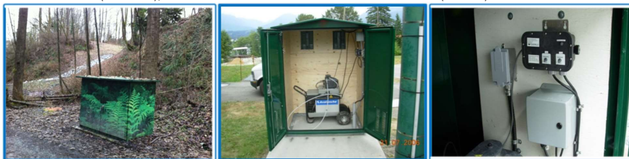
FIGURE 10.3 CSO INFRASTRUCTURE: SAMPLING KIOSK (LEFT), KIOSK WITH AUTOSAMPLER (CENTER), SAMPLER COMMUNICATION ELECTRONICS (RIGHT)
