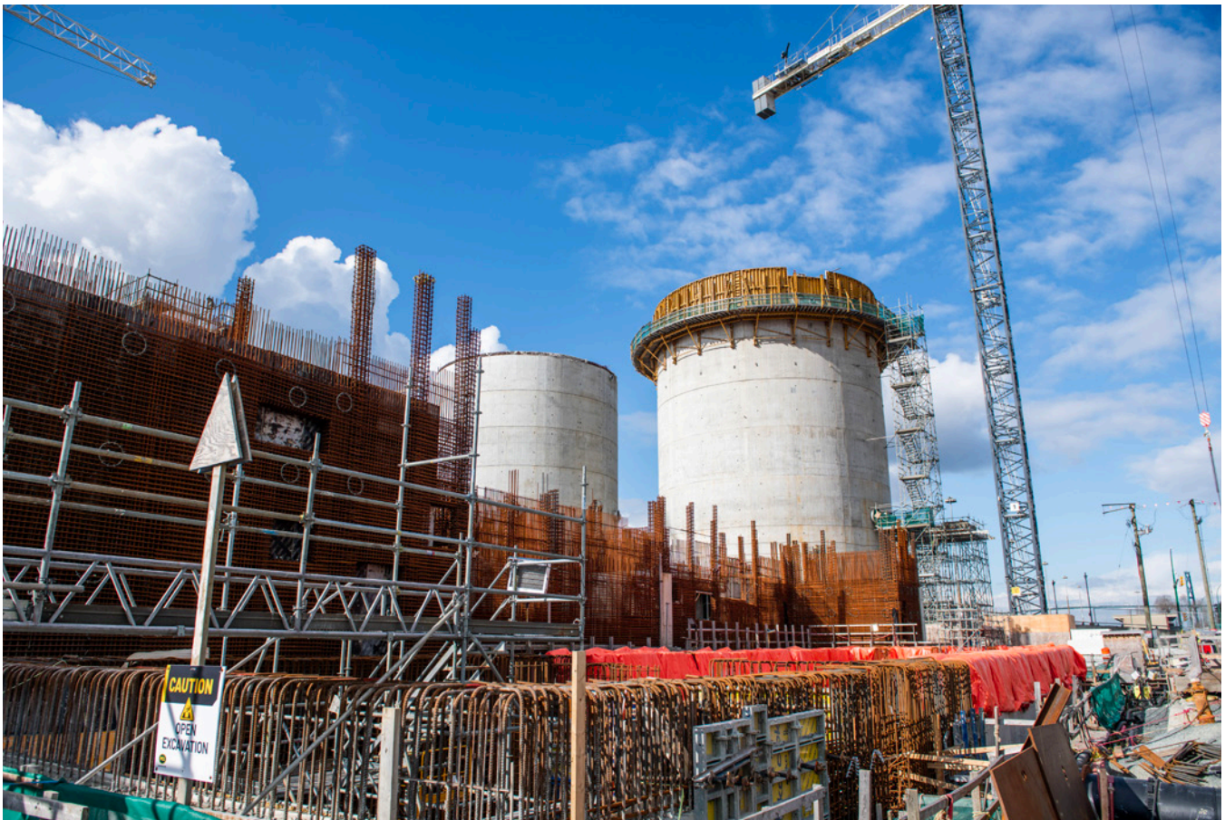
Digesters under construction at west end of treatment plant site
