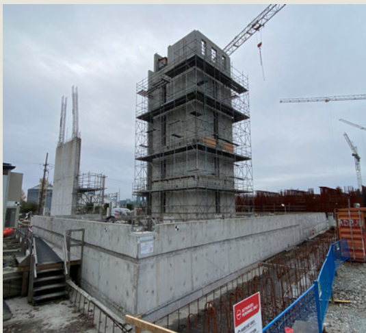
PCL construction progress: concrete foundation for the operations & maintenance building (L), digester roof concrete pours (R)
