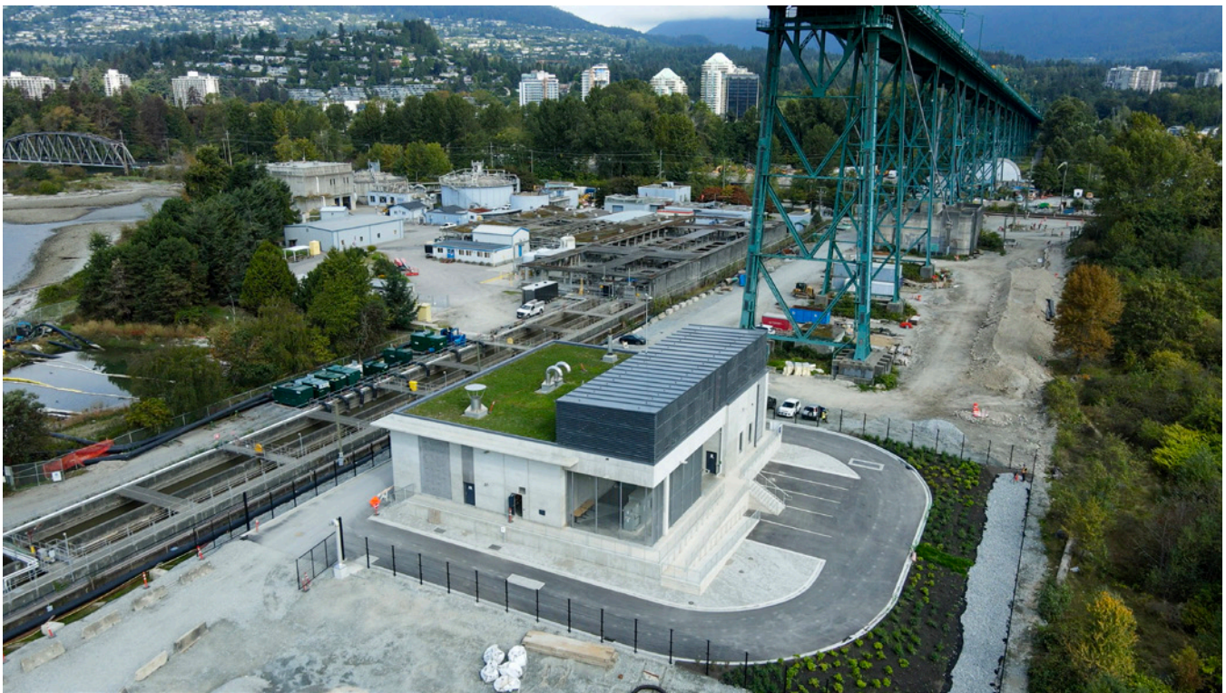
First Narrows Pump Station
