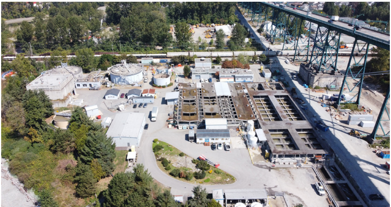
Lions Gate Wastewater Treatment Plant
