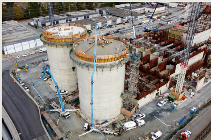
PCL construction progress: concrete foundation for the operations & maintenance building (L), digester roof concrete pours (R)
