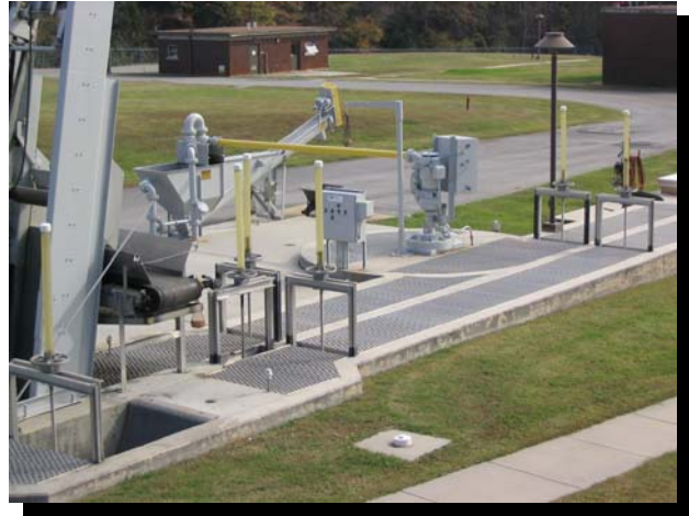
Typical Vortex Grit Removal System
