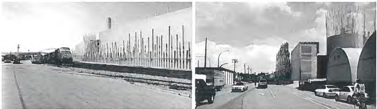
(top) View of Operations and Maintenance building from corner of Pemberton and 1st St (bottom left) View of Southwest end of plant from McKen Rd (bottom right) View of digesters and screening building from further west along 1st St
