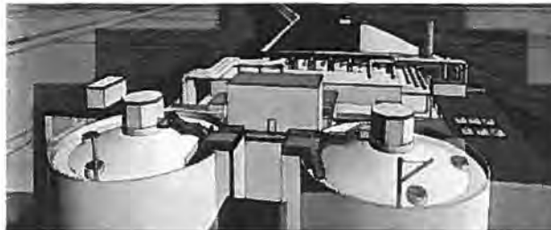
View east, across digesters to solids management and odour control
