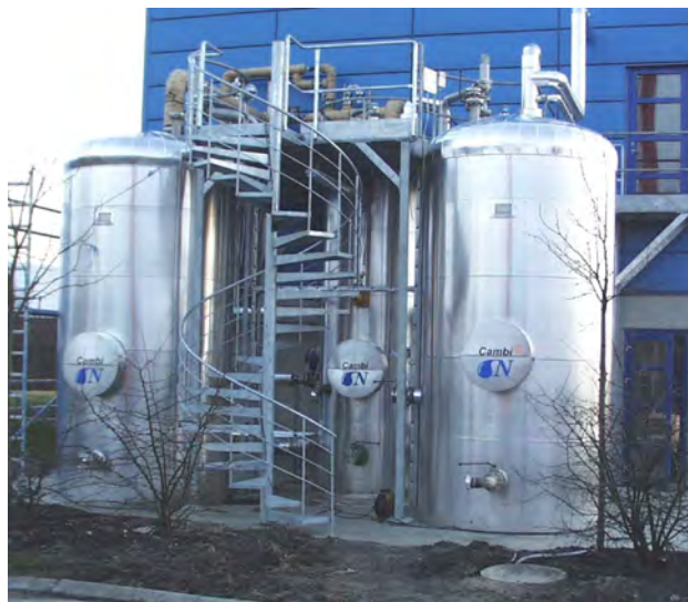
FIGURE 7.4 THERMO HYDROLYSIS (SOURCE: CAMBI®)
