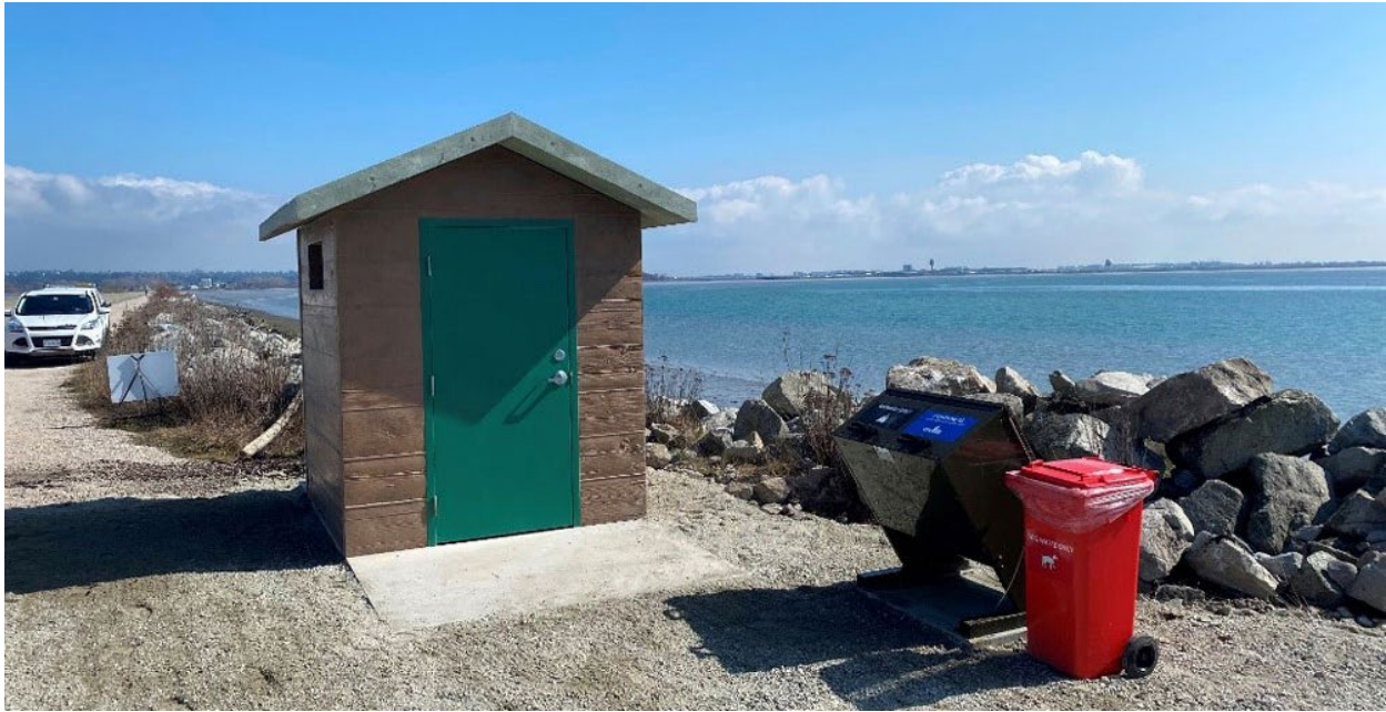
New public pit toilet located at the mid-point of the Iona Jetty.
