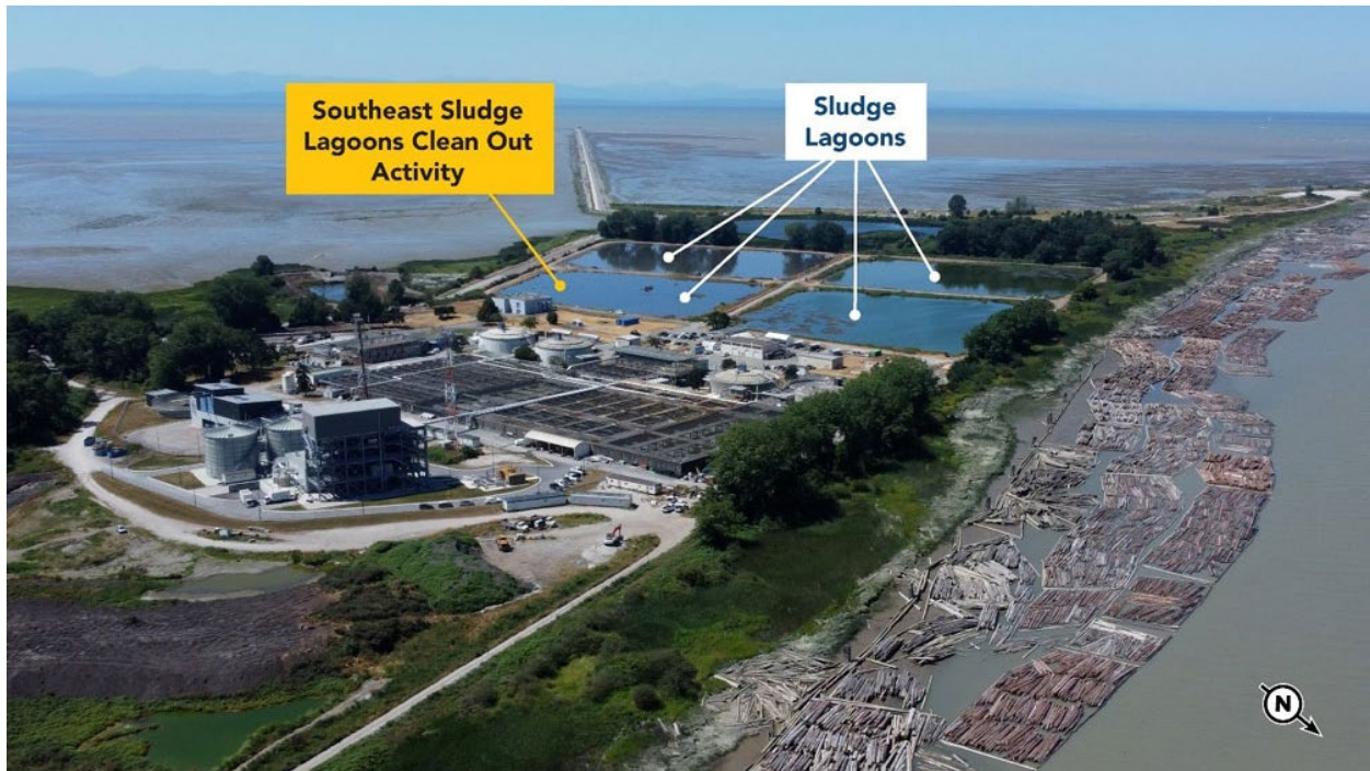
Location of the Iona Island Wastewater Treatment Plant treated sludge lagoons.
