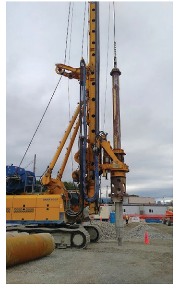
DRILLING AND VIBRATION OF GRANULAR MATERIAL TO INSTALL STONE COLUMNS
