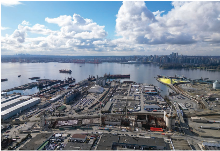
NORTH SHORE WASTEWATER TREATMENT PLANT PROJECT SITE, ADJACENT TO THE BURRARD INLET
