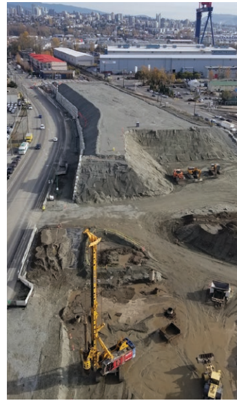
PRELOADING SAND ON THE EAST SIDE OF THE SITE
