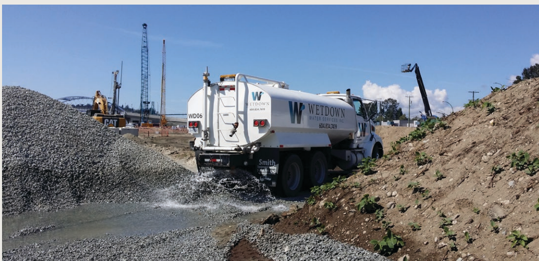
Metro Vancouver implementing dust control measures
