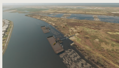
Site 2 – Adjacent to the Construction Laydown Area
