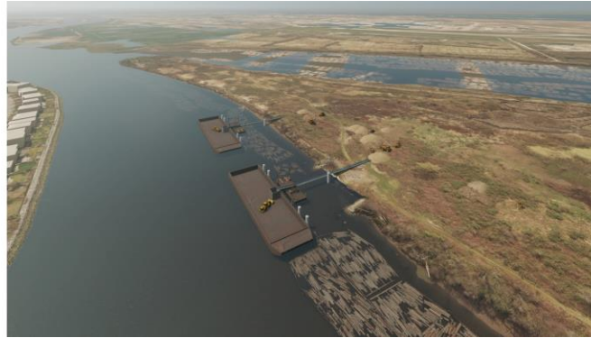
Site 2 – Adjacent to the Construction Laydown Area
