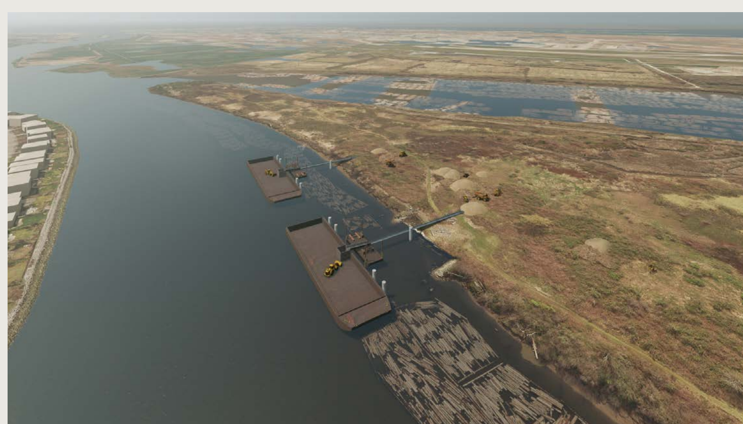
Site 2 – Adjacent to the Construction Laydown Area
