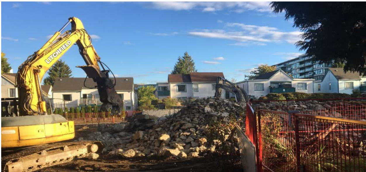
Figure 4: Deconstruction at Heather Place
