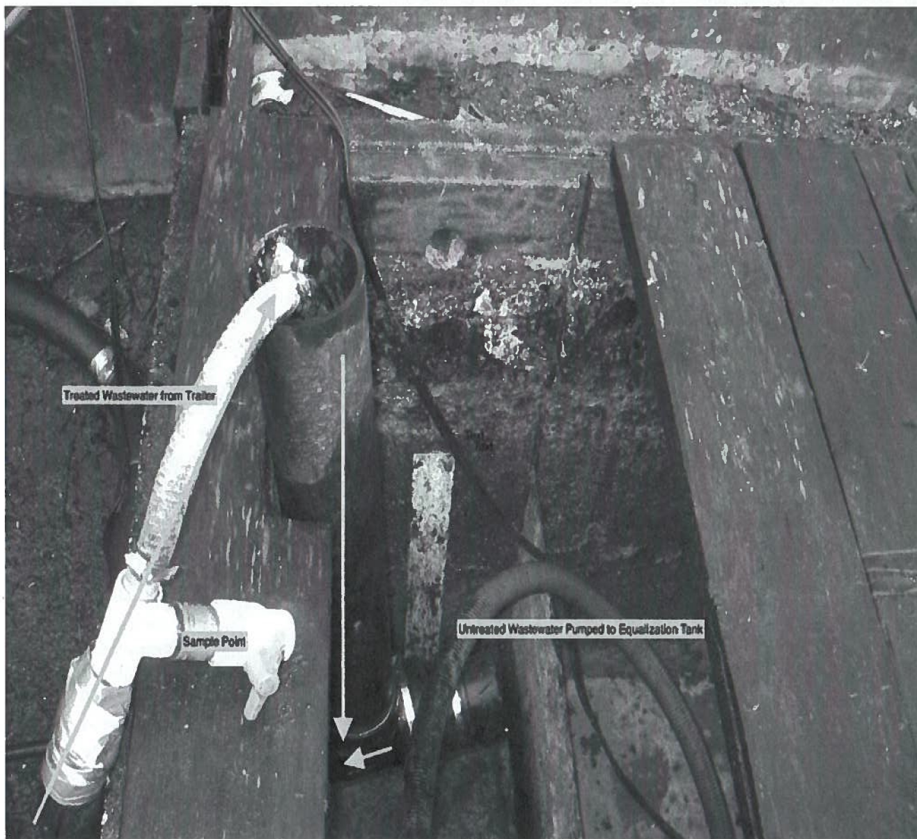
Photograph of Sample Point 1:
