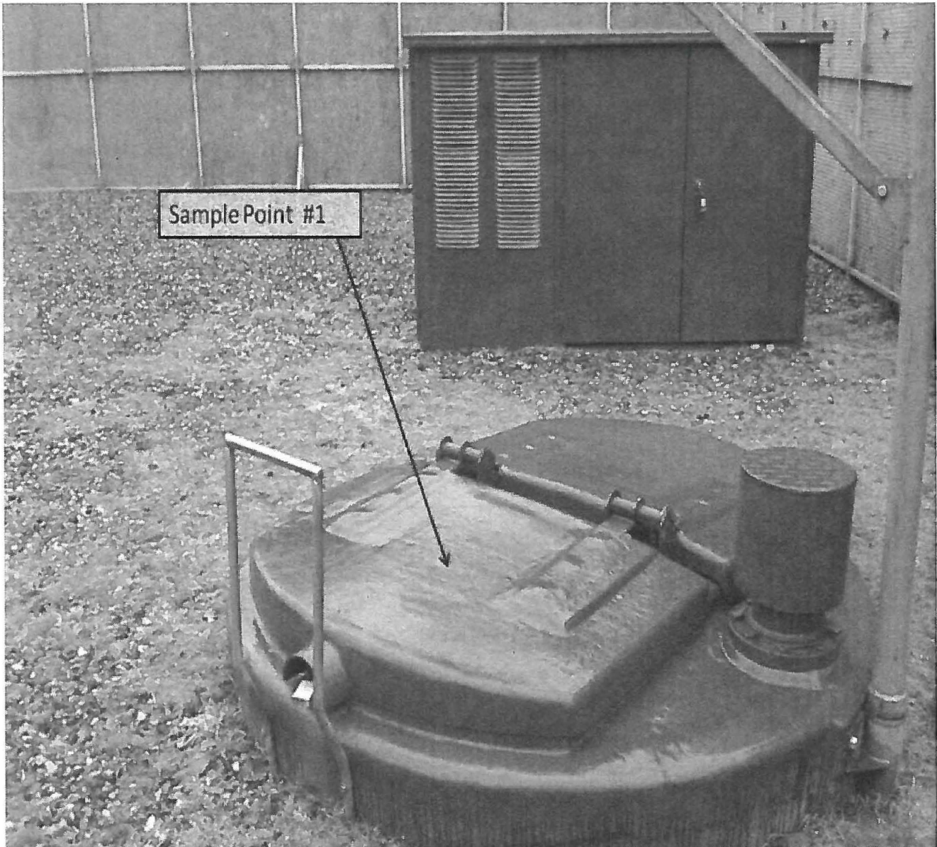
Photograph of Sample Point 1:
